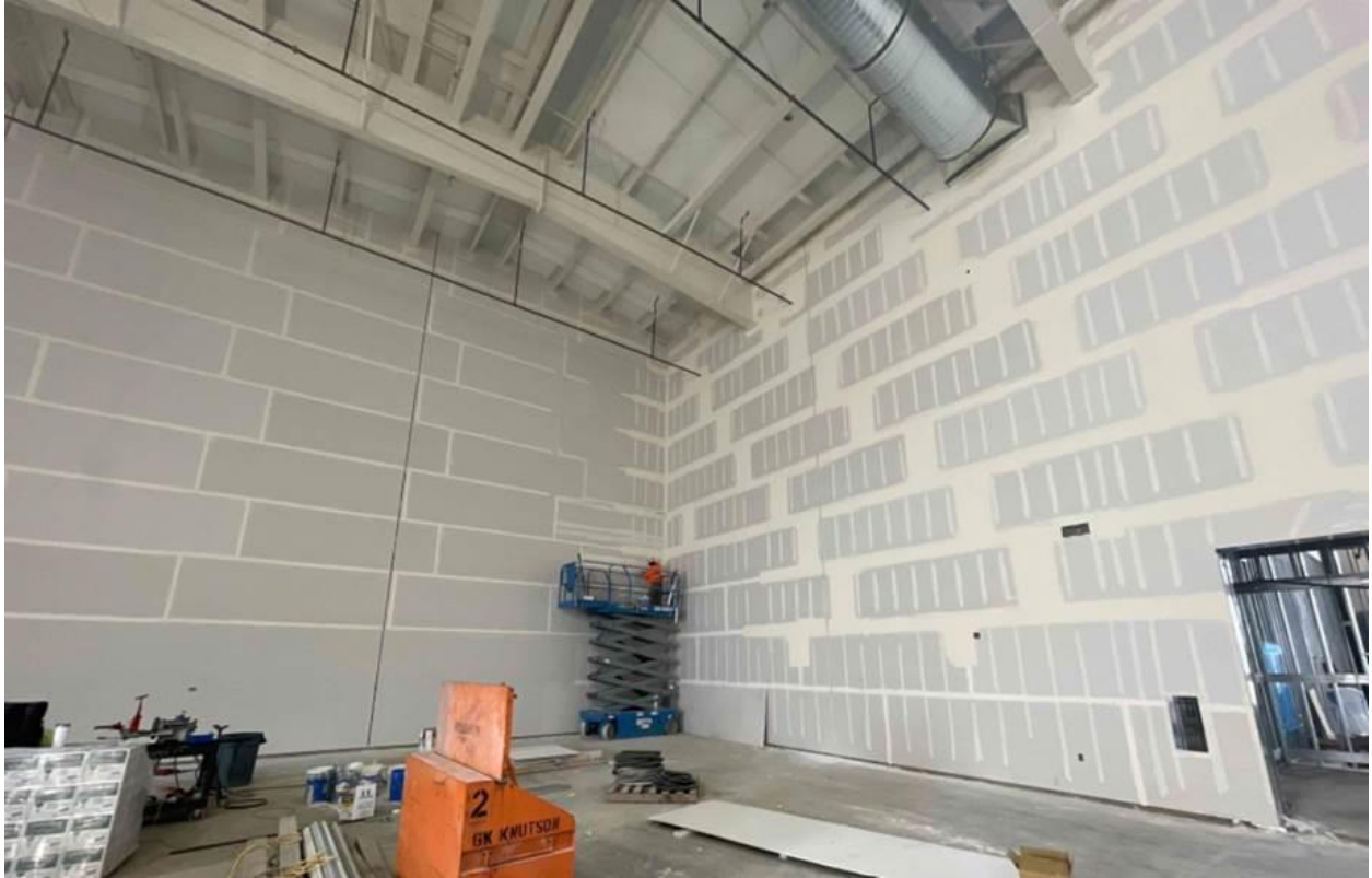
Sheetrock taping and mudding in the Main Gym
