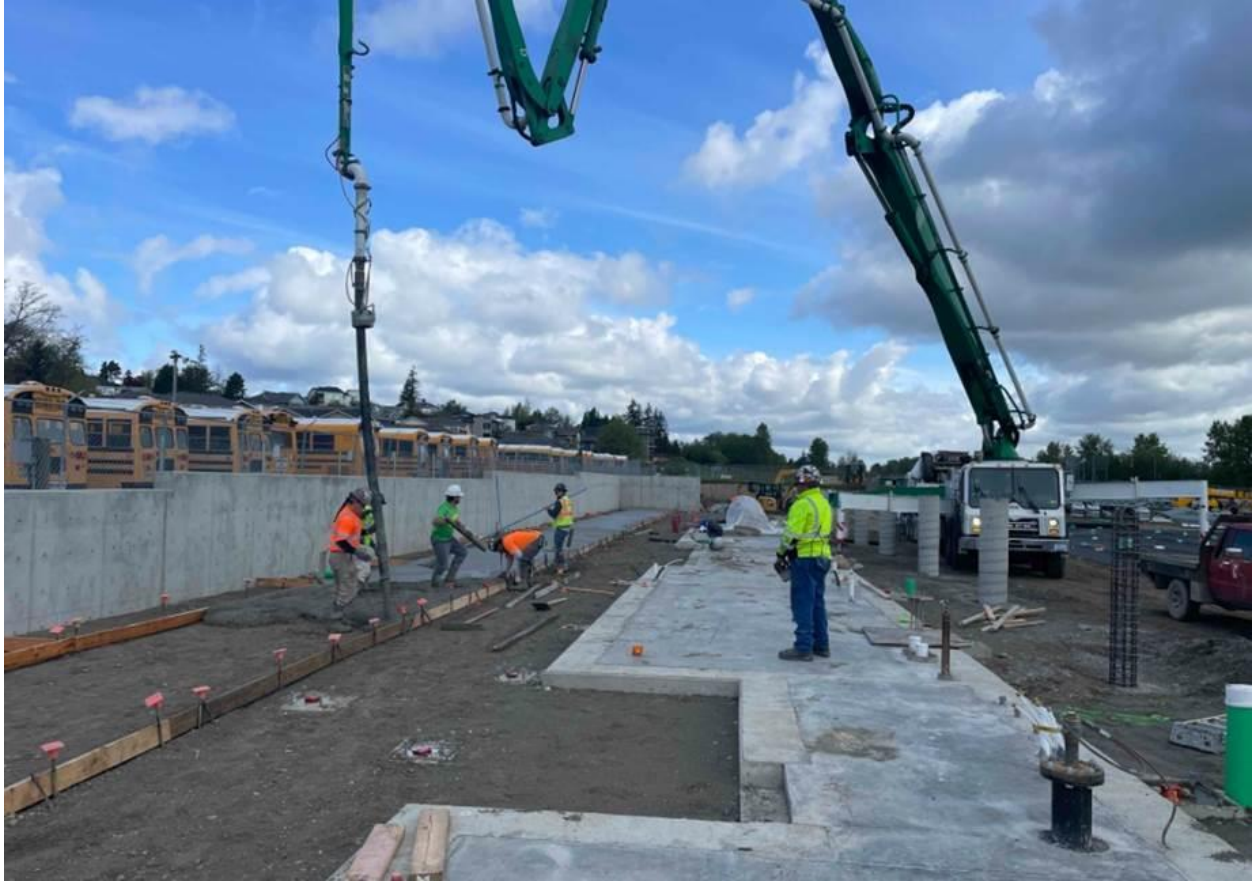
Hardscape pouring around the Grandstands area
