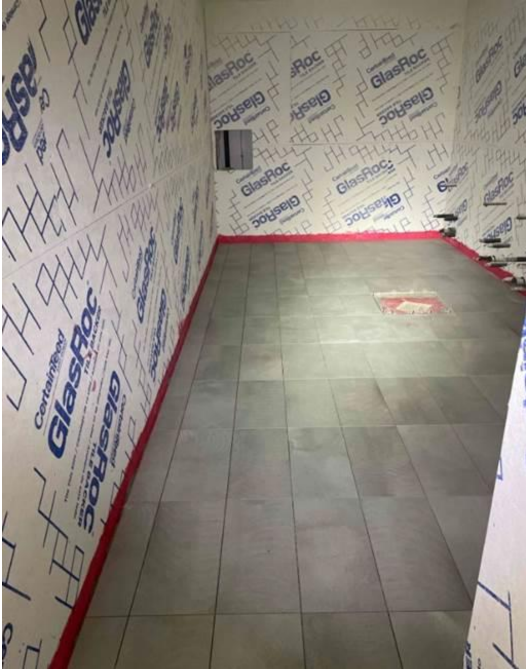
Bathroom floor tile installation in the Academic Wing
