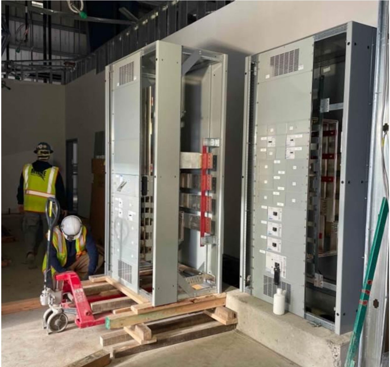
Main electrical panel installation in the Athletic Wing
