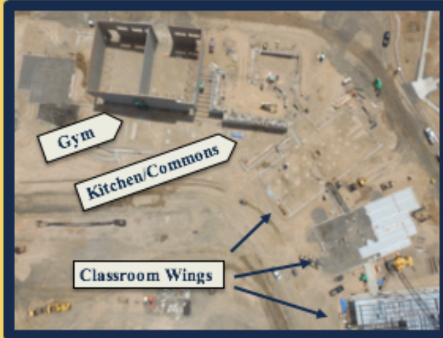
Aerial View Highland Middle School 3515 W. Hawthorne Rd., Spokane, WA 99208
