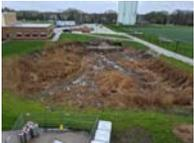
Site work has started on new pool construction. Load tests for micro-piers have been completed, and foundation work for pool to begin the week of May 4. Meeting was held with donors to discuss signage and donor acknowledgment. In development.
