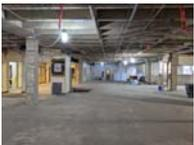
Demolition has been completed. Above ceiling MEP rough-in is ongoing. Wall layout and framing and CMU wall construction began on May 5. Project was started two weeks ahead of schedule.
