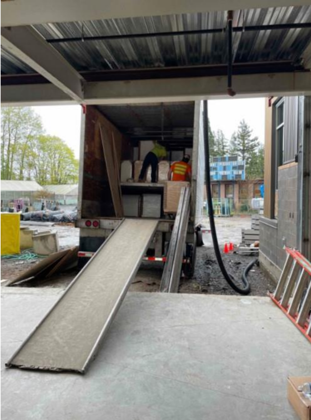
Cabinets for the first floor of the Academic Wing being delivered
