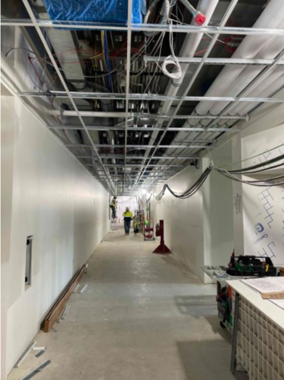
Ceiling grid being installed in the Academic Wing's first floor
