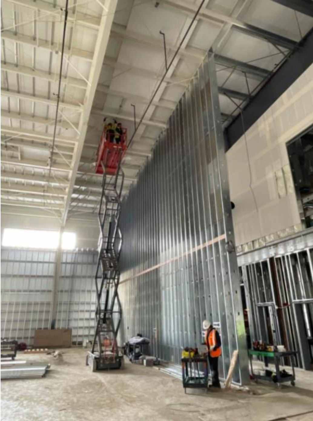
Crews installing wall framing in the Main Gym
