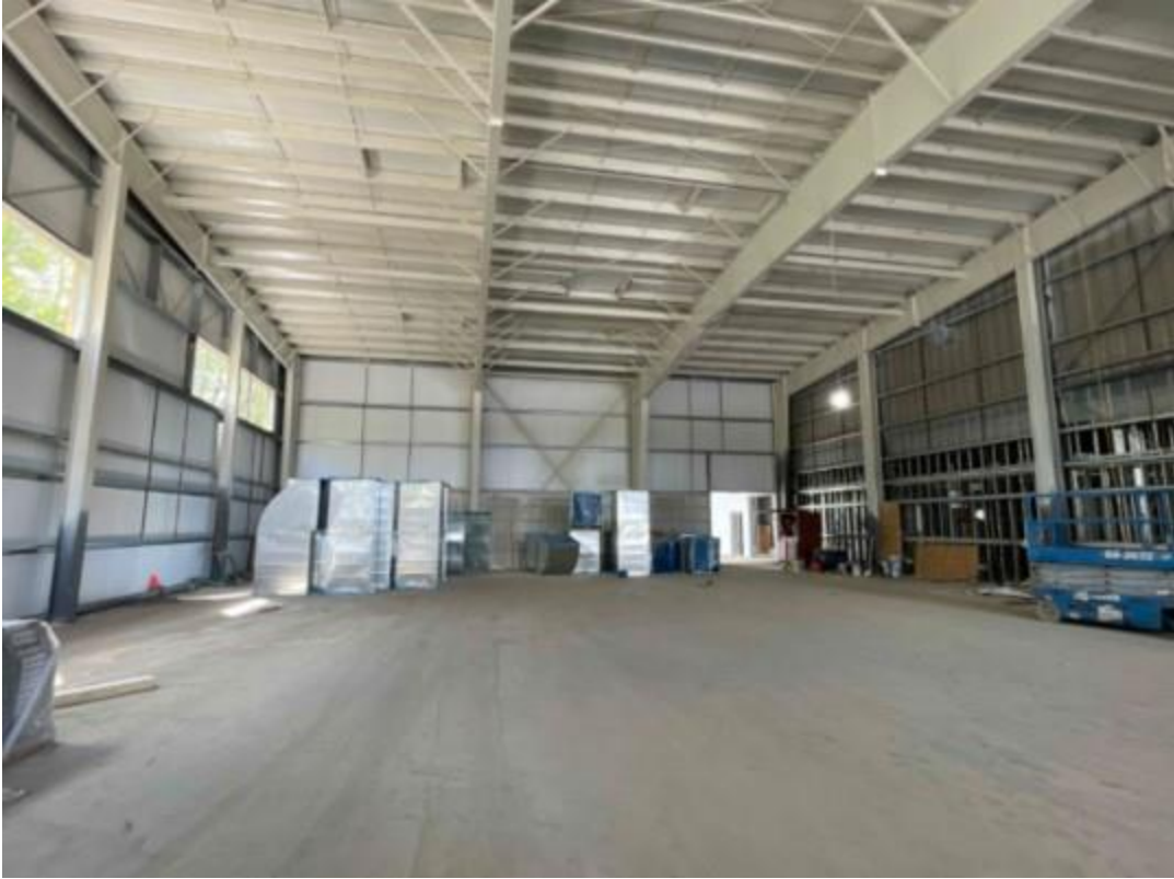
Completed overhead painting in the Auxiliary Gym
