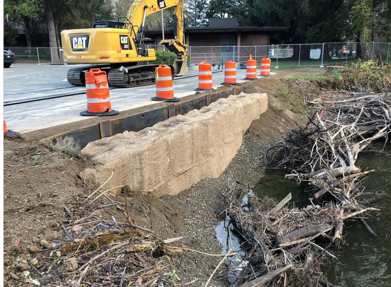
Temporary stream bank protection work completed
