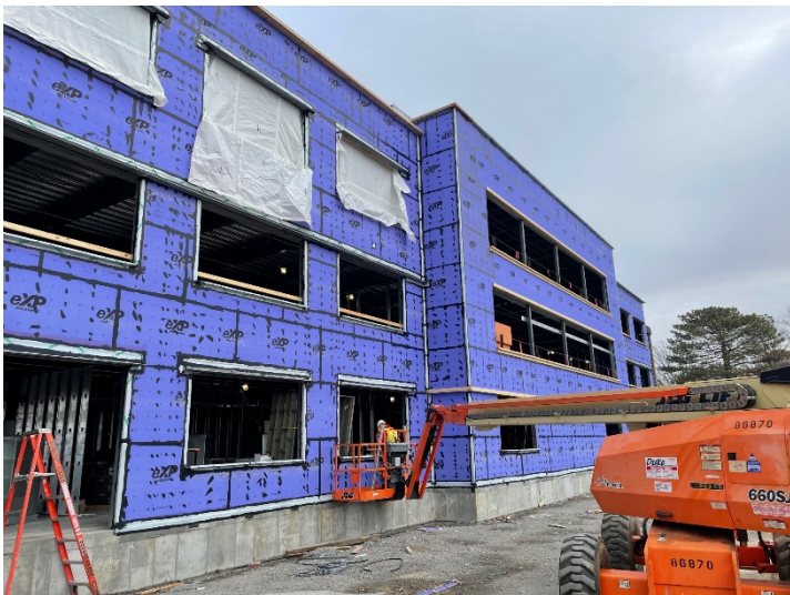
Air Barrier Install
