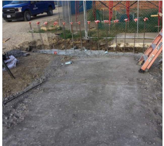
Retaining Wall Footing
