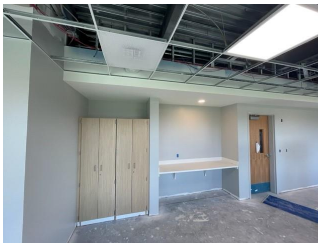
Ceiling Grid and Counter Tops Installed
