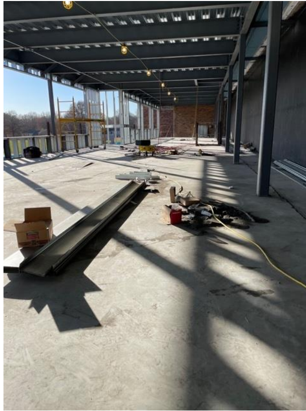
2 nd Floor Slab On Deck
