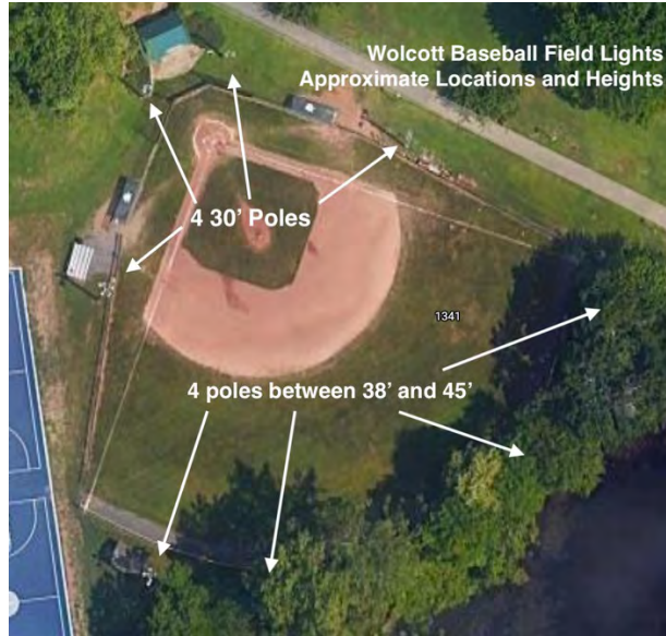
Figure 2: Existing Wolcott Light Pole Locations and Heights
