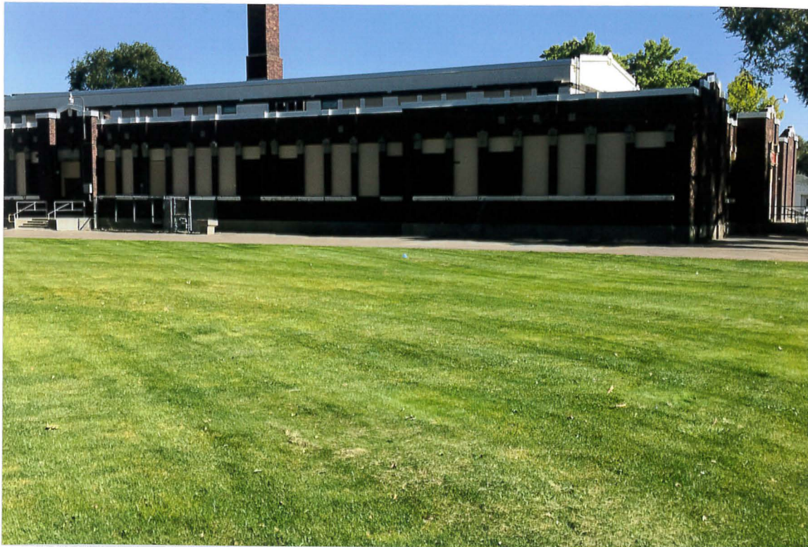
1 and 2 - View of the North side of the Original Building. Fremont Street side.
