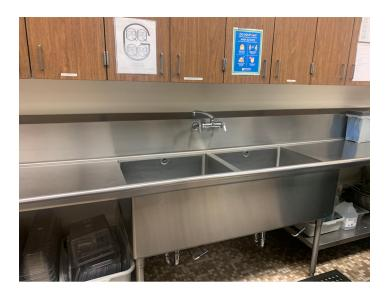
Under prep sink that is currently directly drained to sanitary. Scope is to install a hub drain under the sink and indirectly drain the prep sink into the new hub drain to meet code and health department requirements.
