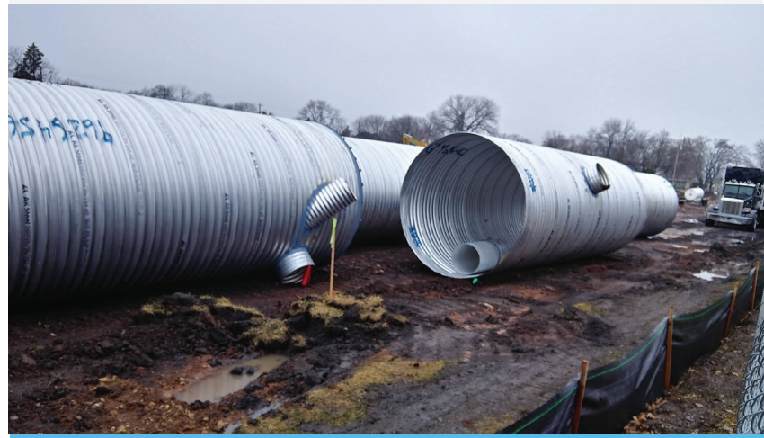
VPMS DRAINAGE CULVERTS AWAITING INSTALLATION
