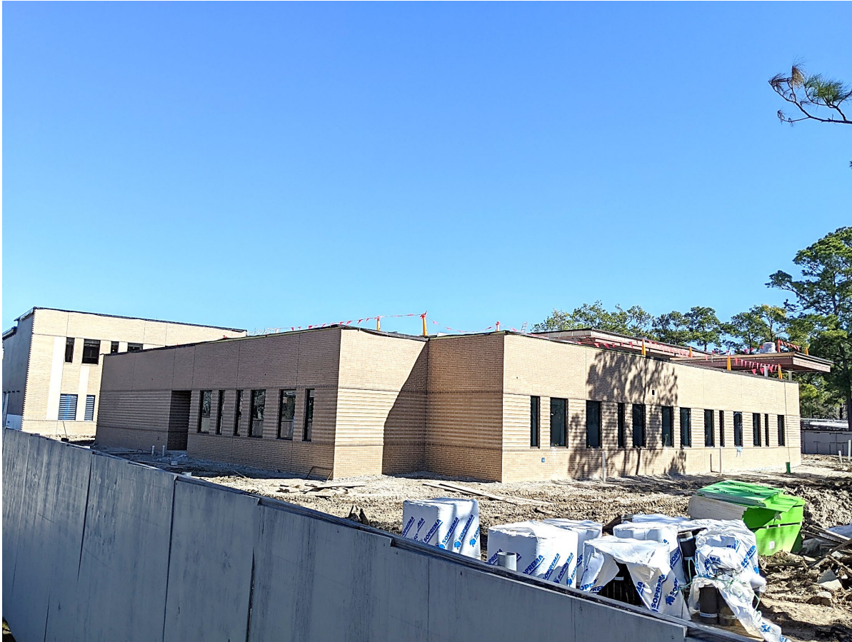
Masonry and glazing progress at Administration and adjacent classroom wing
