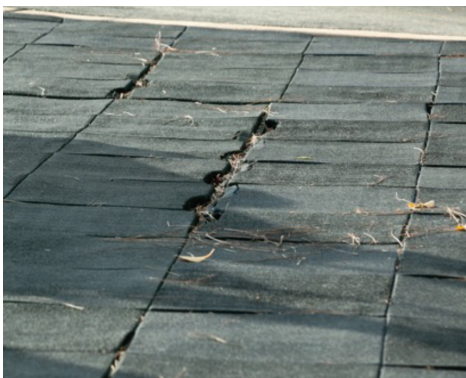
DETERIORATING PLAY MATTING PRIOR TO MEASURE M RENOVATIONS
