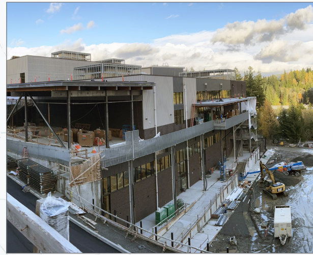
Cougar Mountain Middle School in the Talus Neighborhood under construction, pictured in November 2021.
