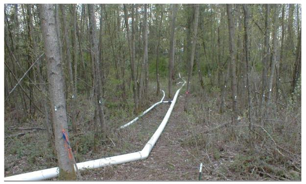
Figure 3 - 26: Manifold and Branches in a Wooded, Vegetated Spray Field
