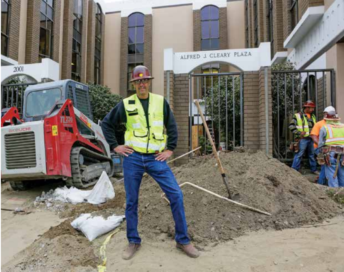
Lloyd Berges supervised the seismic upgrades at SI, with most of the work finishing just before the August quake.
