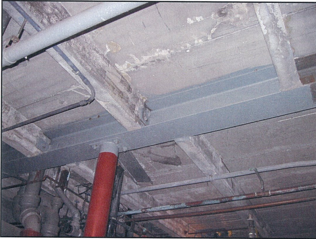
Photo P-9: Bathhouse Concrete Floor Joist Reinforcement Exposed
