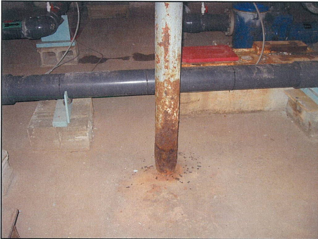
Photo P-7: Bathhouse Column Corrosion
