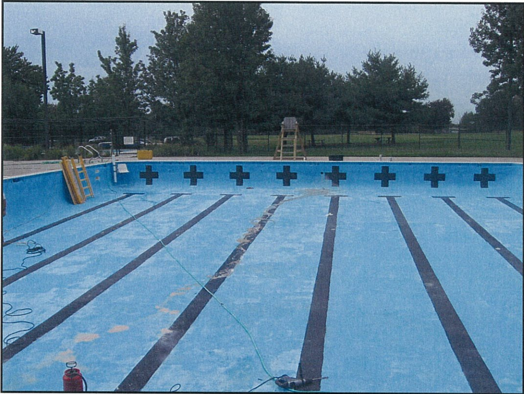
Photo P-3: Exposed Pool Walls and Floor
