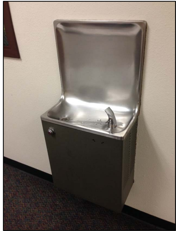
Sample TTS122116-P-DF-15: 15 µg/L initial lead concentration. Drinking fountain above is identified producing elevated lead concentrations.
