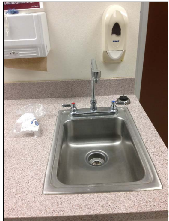
Sample TTS122116-P-KF-10: 2 µg/L initial lead concentration. Same fixture style as CF-34 and KF-27 identified producing elevated lead concentrations.
