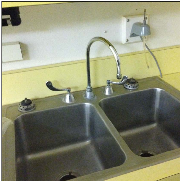
Sample TTS122116-P-KF-28: 41 µg/L initial lead concentration. Fixture style above is identified producing elevated lead concentrations.
