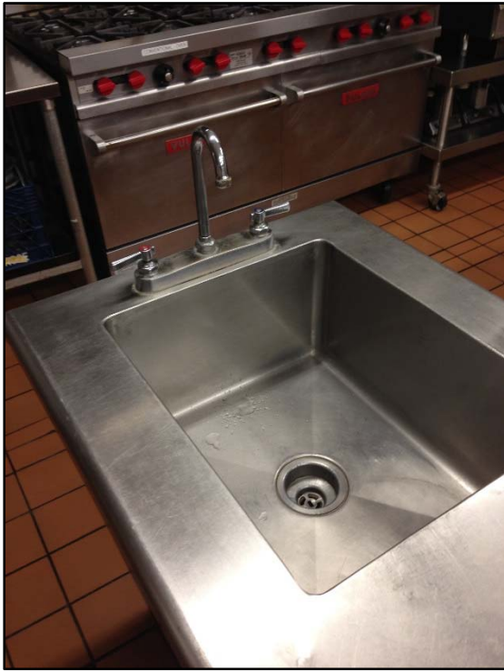
Sample TTS122116-P-KF-05: 23 µg/L initial lead concentration. Fixture style above is identified producing elevated lead concentrations.
