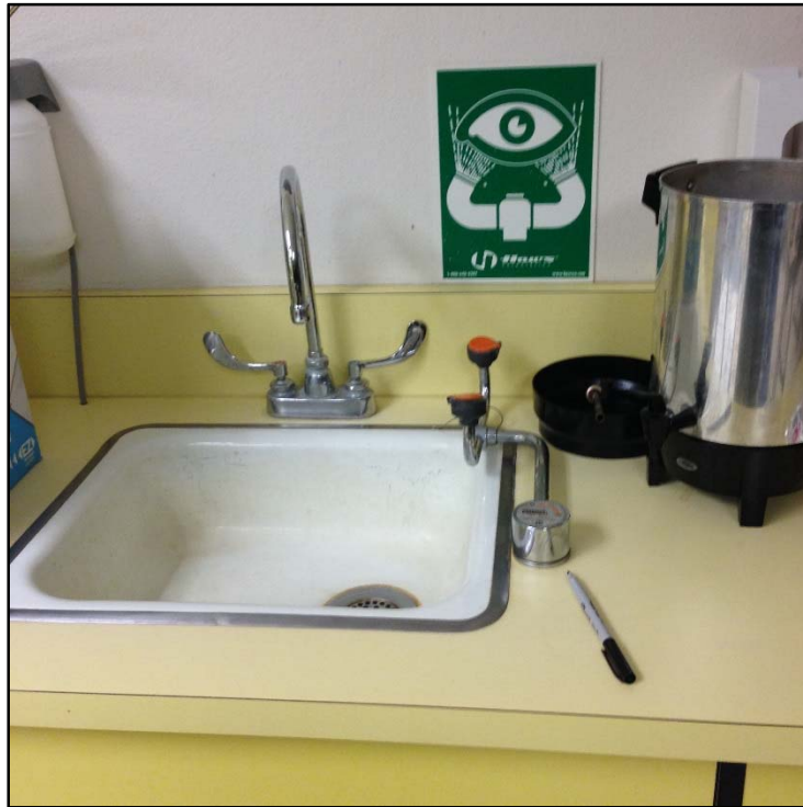
Sample TTS122116-P-KF-26: 30 µg/L initial lead concentration. Fixture style above is identified producing elevated lead concentrations.
