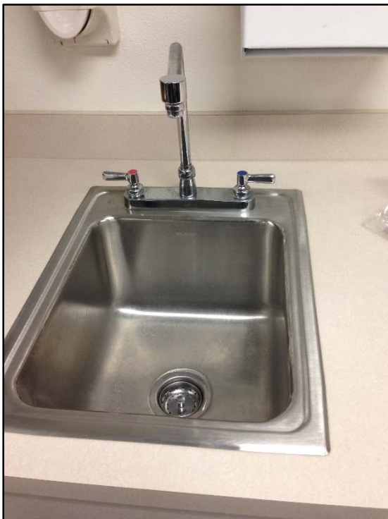
Sample TTS122116-P-CF-34: 28 µg/L initial lead concentration. Fixture style above is identified producing elevated lead concentrations.
