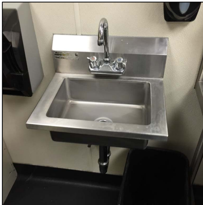
Sample 122116-SVE-P-KF-13: 2 µg/L initial lead concentration. Same fixture style as initial sample with elevated lead concentration.
