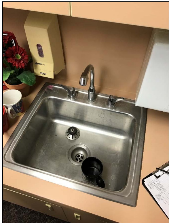
Sample RVE122116-P-CF-26: 13 µg/L initial lead concentration. Fixture style above is identified producing elevated lead concentrations.
