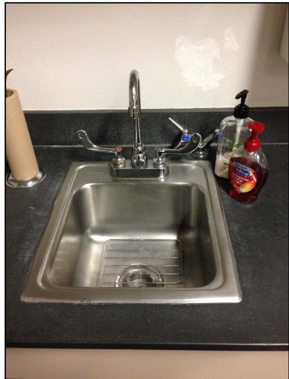
Sample AE122216-P-CF-07: 12 µg/L initial lead concentration. Same fixture style as classroom faucets with elevated lead concentrations.
