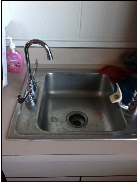
Sample HMS122116-P-CF-14: 19 µg/L initial lead concentration. Faucet above is identified producing elevated lead concentrations.
