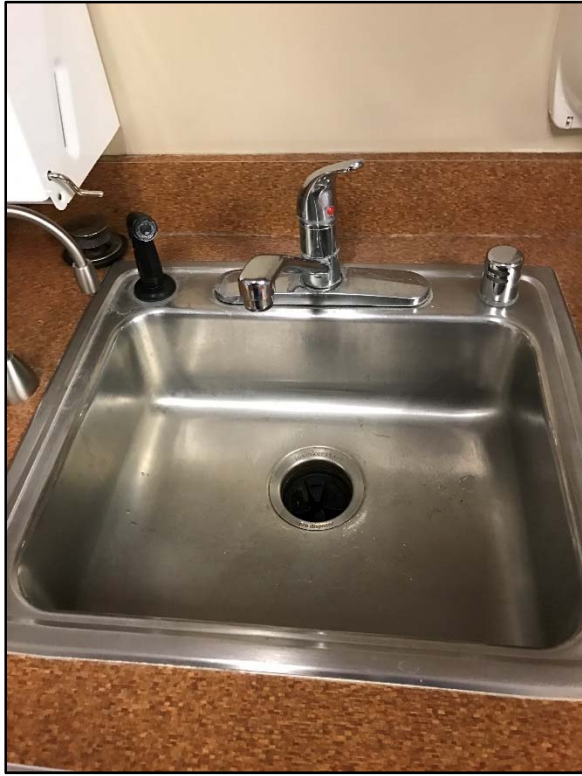
Sample CWE122116-P-OF-11: 25 µg/L initial lead concentration. Fixture style above is identified producing elevated lead concentrations.
