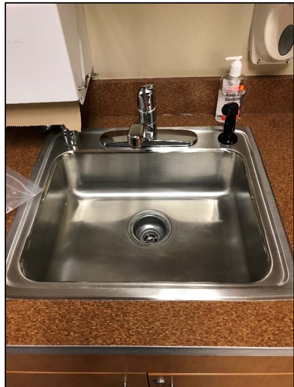
Sample CWE122116-P-OF-11: 4 µg/L initial lead concentration. Same fixture style as initial sample with elevated lead concentration.
