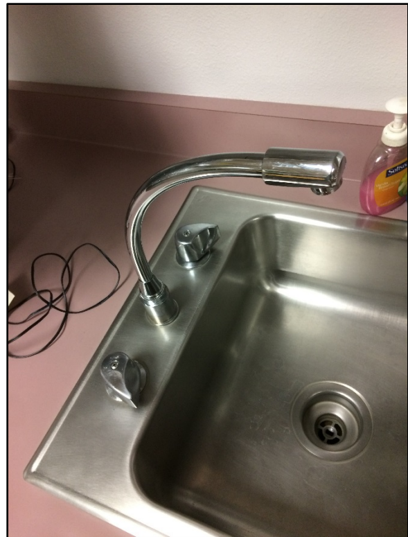
Sample HHH122216-P-CF-17: 7 µg/L initial lead concentration. Same fixture style as initial sample identified with an elevated lead concentration.
