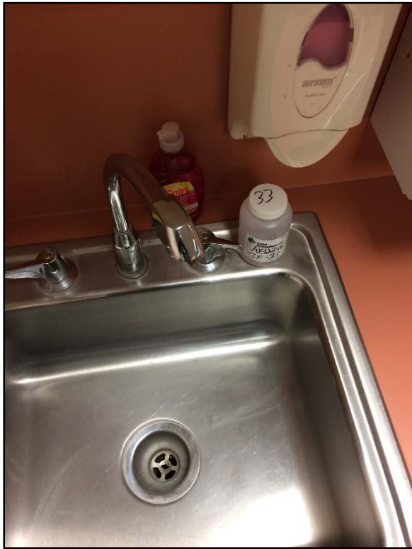
Sample AE122216-P-CF-33: 15 µg/L initial lead concentration. Fixture style above is identified producing elevated lead concentrations.
