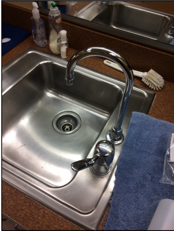
Sample CCE122216-P-OF-08: 49 µg/L initial lead concentration. Fixture style above is identified producing elevated lead concentrations.
