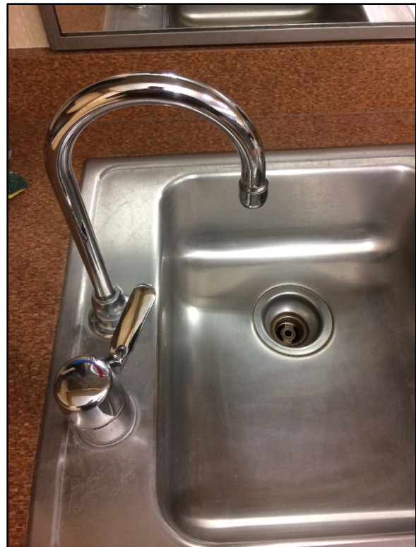
Sample CCE122216-P-CF-23: <1.0 µg/L initial lead concentration. Same fixture style as initial sample with elevated lead concentration.
