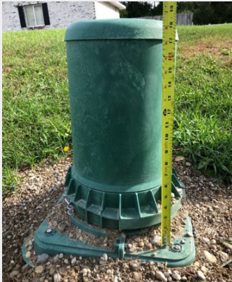
Ground Level Closure Pedestal Size: 18.5 inches tall Number of pedestals in Oakwood: Approximately 200
