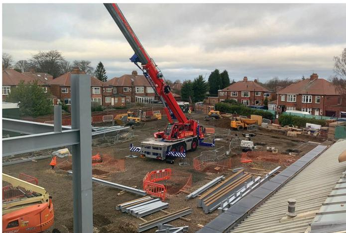
**With foundation works now completed on our North End Development, principal contractor Tolent has begun erecting the steel frame.**
