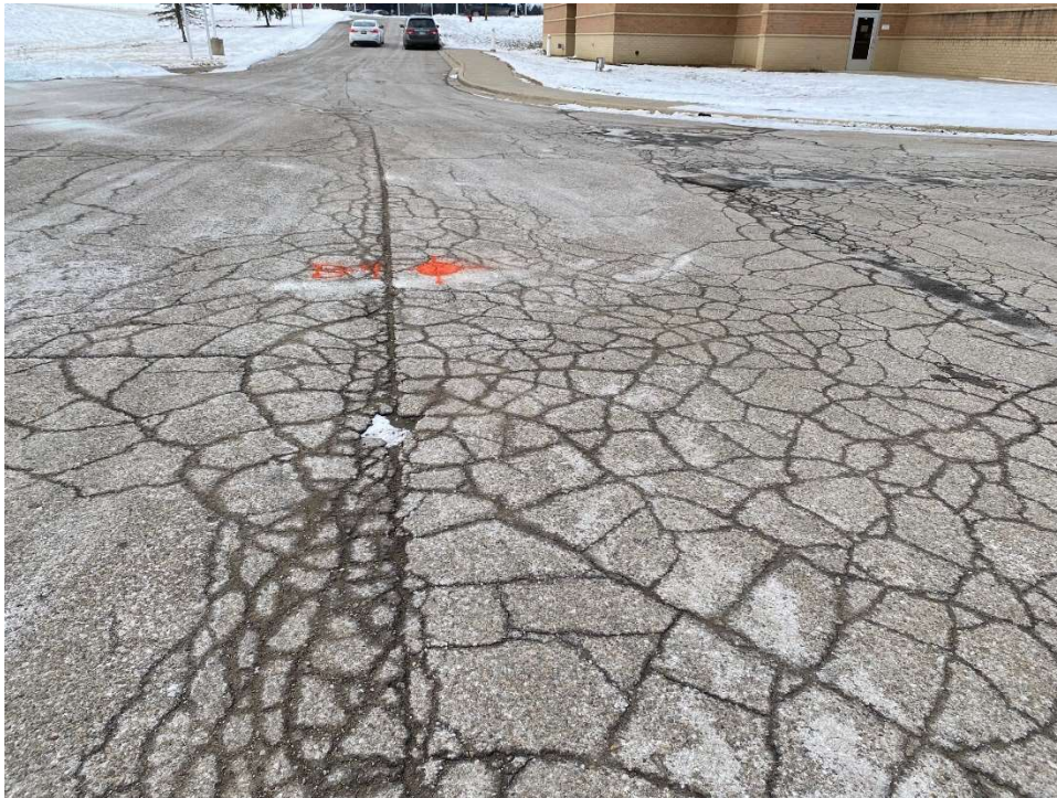
Photograph No. 4: High severity block and fatigue cracking at Dexter High School near boring B-04. View to the northwest.
