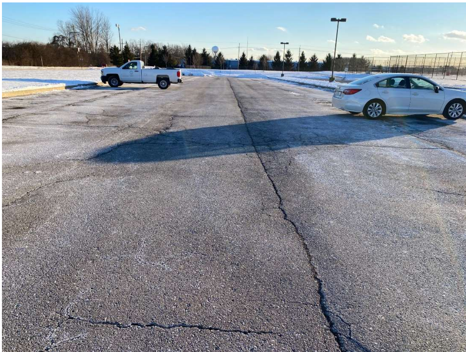
Photograph No. 20: Moderate severity fatigue, block, and transverse and longitudinal cracking at Mill Creek Middle School southwest parking lot. View to the south.
