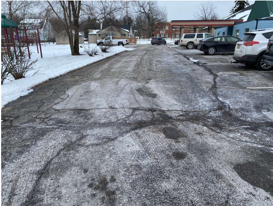
Photograph No. 9: Moderate to high severity block and fatigue cracking with surface patching at Jenkins Early Education Center near boring B-09. View to the west.
