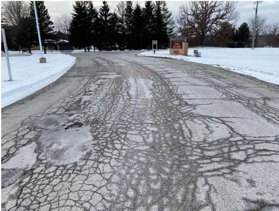
Photograph No. 6: High severity block and fatigue cracking with cold patching at Dexter High School near boring B-06. View to the west.
