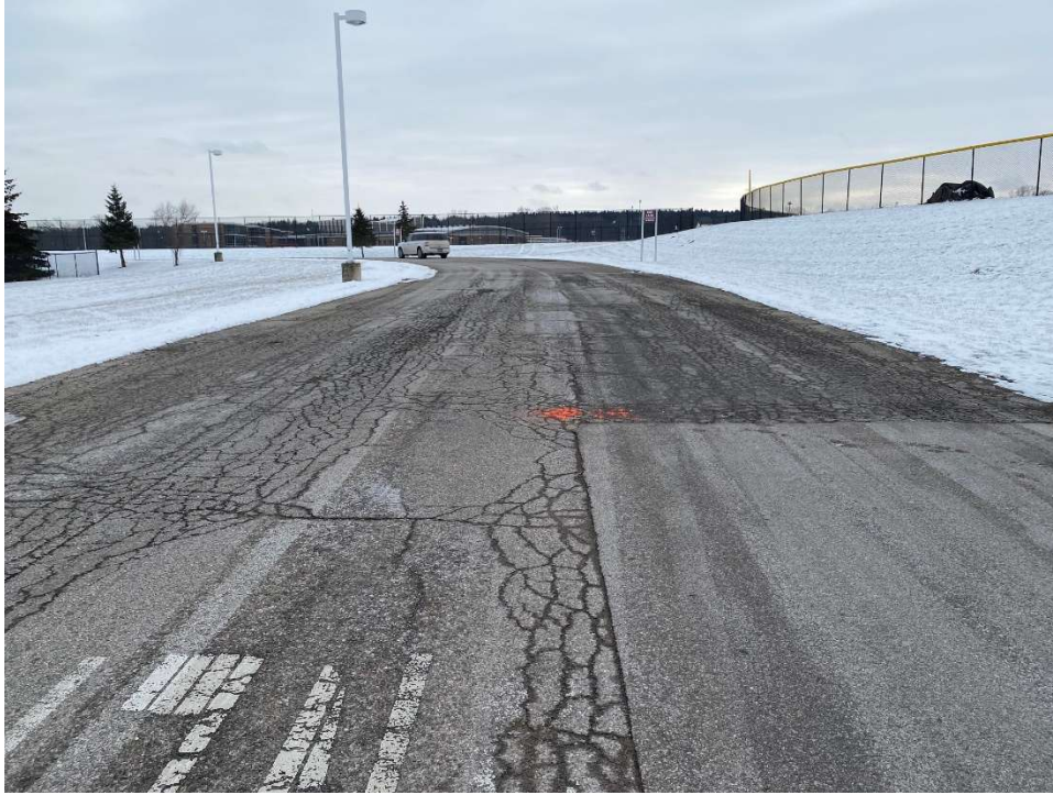
Photograph No. 1: High severity block and fatigue cracking with surface patching at Dexter High School near boring B-01. View to the south.
