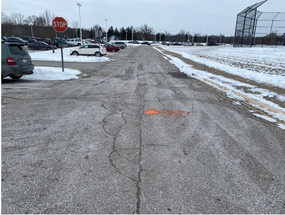
Photograph No. 3: Moderate to high severity transverse, longitudinal, and edge cracking at Dexter High School near boring B-03. View to the west.
