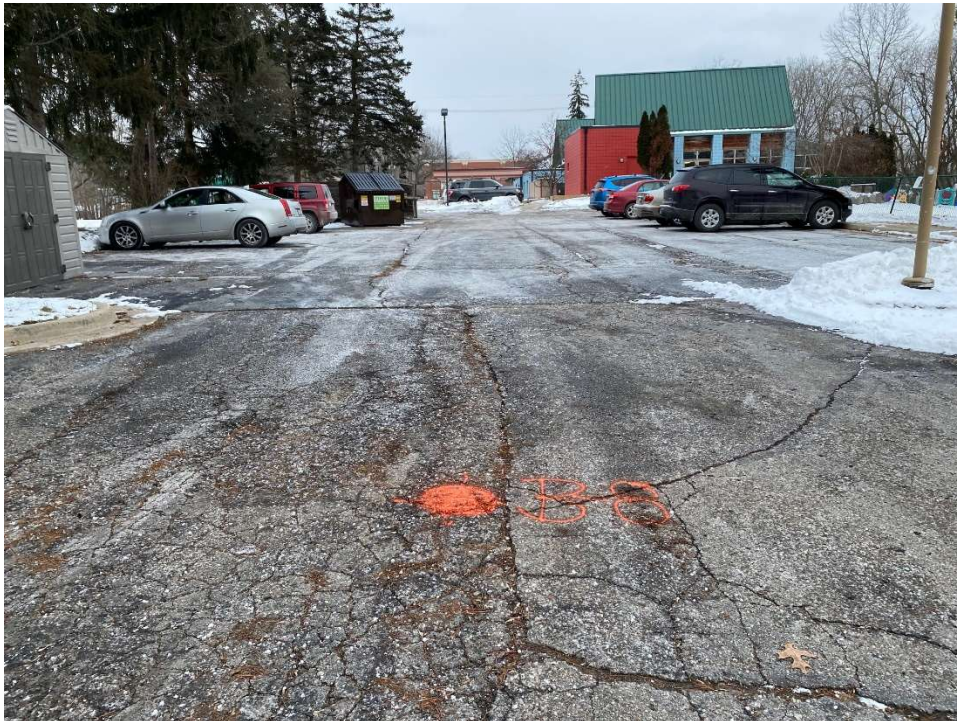
Photograph No. 8: Moderate to high severity block and fatigue cracking at Jenkins Early Education Center near boring B-08. View to the west.
