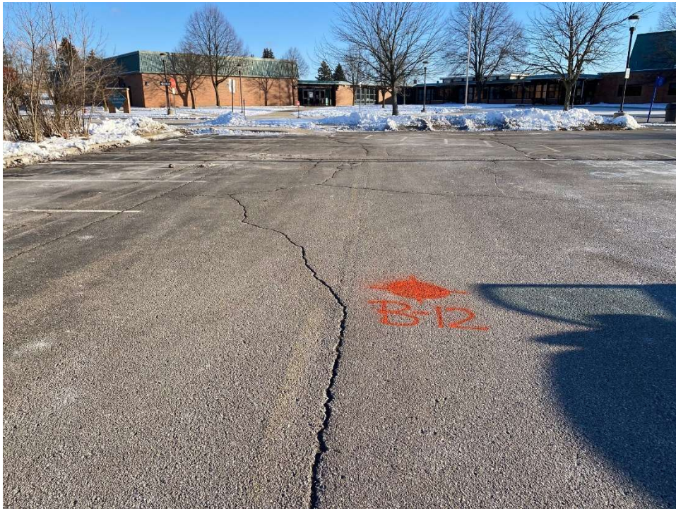
Photograph No. 12: Low to moderate severity longitudinal and transverse cracking with at Wylie Elementary School near boring B-12. View to the southeast.
