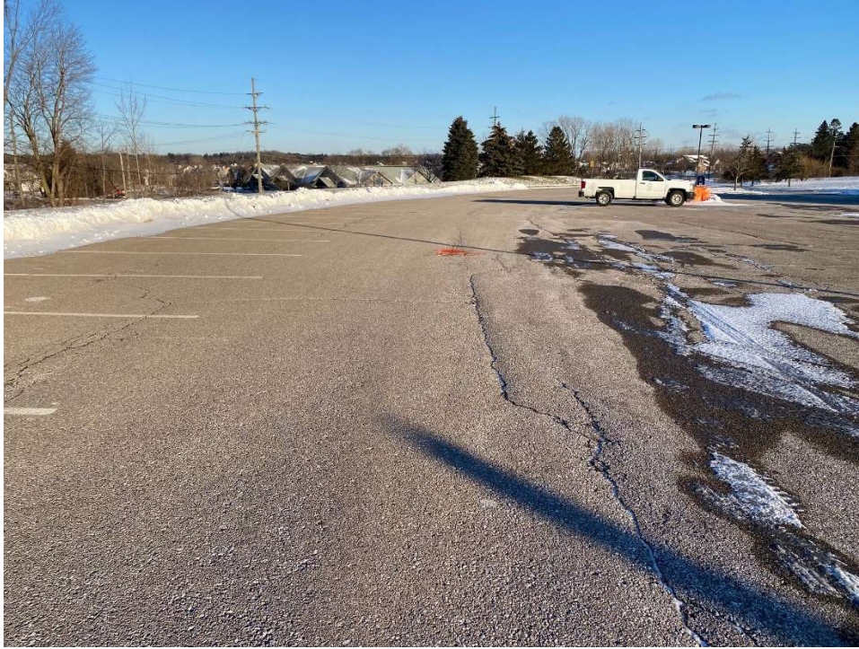
Photograph No. 17: Low to moderate severity transverse and longitudinal cracking at Mill Creek Middle School northeast parking lot near boring B-17. View to the east.
