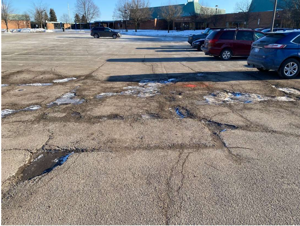
Photograph No. 11: Moderate to high severity fatigue, transverse, and longitudinal cracking with cold patching with at Wylie Elementary School near boring B-11. View to the southeast.
