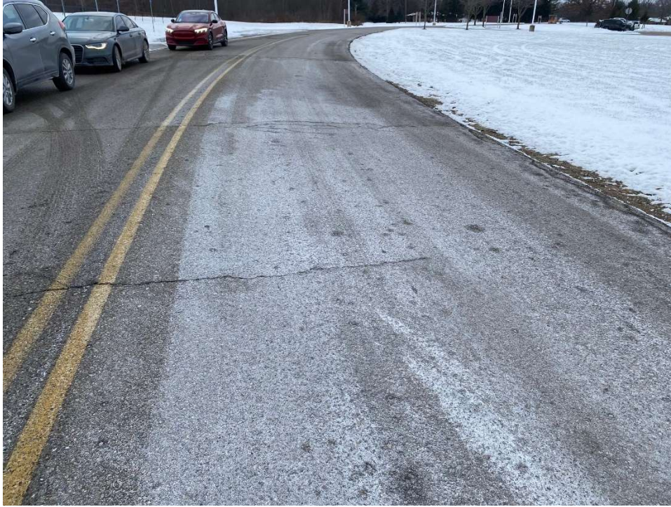
Photograph No. 5: Low severity transverse cracking at Dexter High School near boring B-05. View to the west.
