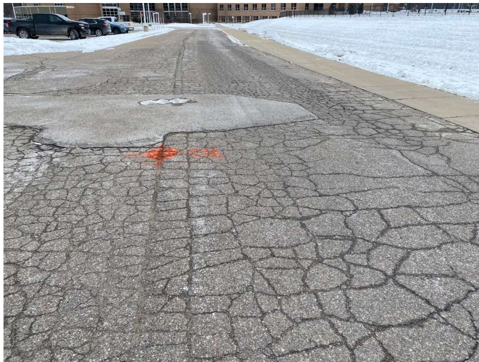
Photograph No. 2: High severity block and fatigue cracking with surface patching at Dexter High School near boring B-02. View to the south.
