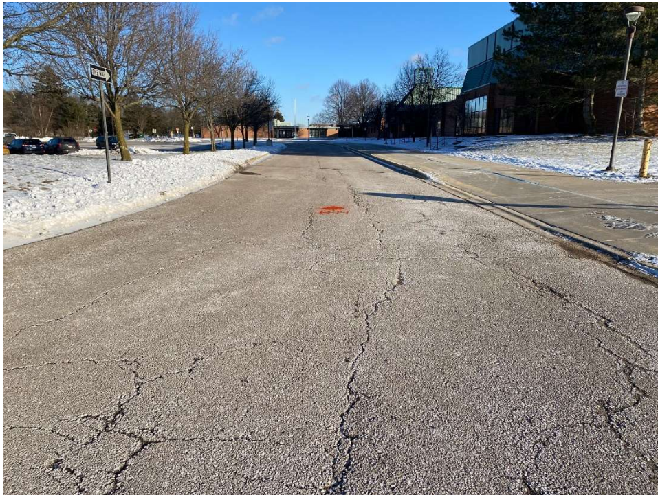
Photograph No. 14: Low to moderate severity longitudinal and transverse cracking with at Wylie Elementary School near boring B-14. View to the east.
