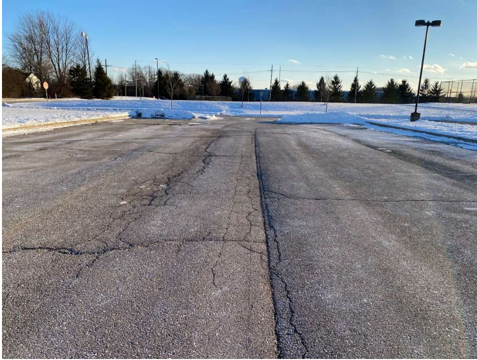
Photograph No. 19: Moderate to high severity fatigue, block, and transverse and longitudinal cracking at Mill Creek Middle School southwest parking lot. View to the south.
