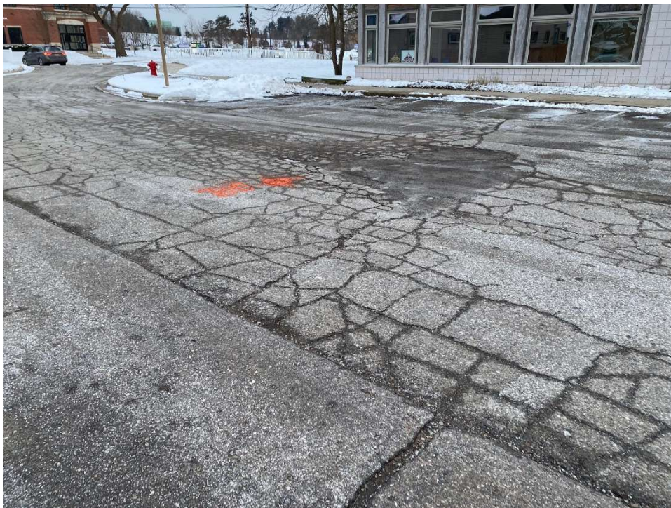
Photograph No. 10: High severity block and fatigue cracking with cold patching at Jenkins Early Education Center near boring B-10. View to the southwest.
