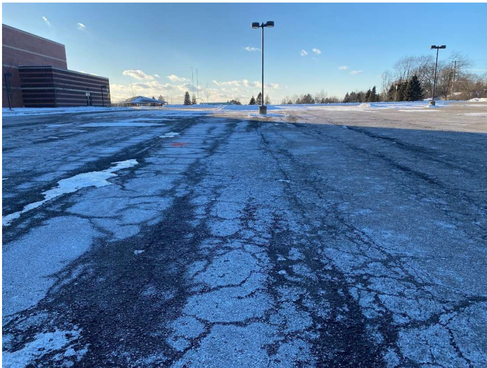
Photograph No. 16: Moderate to high severity fatigue, block, and transverse and longitudinal cracking at Mill Creek Middle School northeast parking lot near boring B-16. View to the west.
