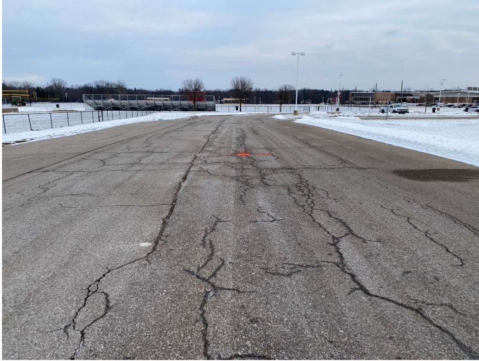
Photograph No. 7: Moderate to high severity transverse, longitudinal, and fatigue cracking at Dexter High School near boring B-07. View to the west.
