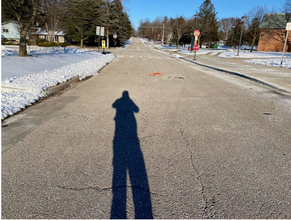
Photograph No. 13: Low severity longitudinal and transverse cracking with at Wylie Elementary School near boring B-13. View to the northeast.
