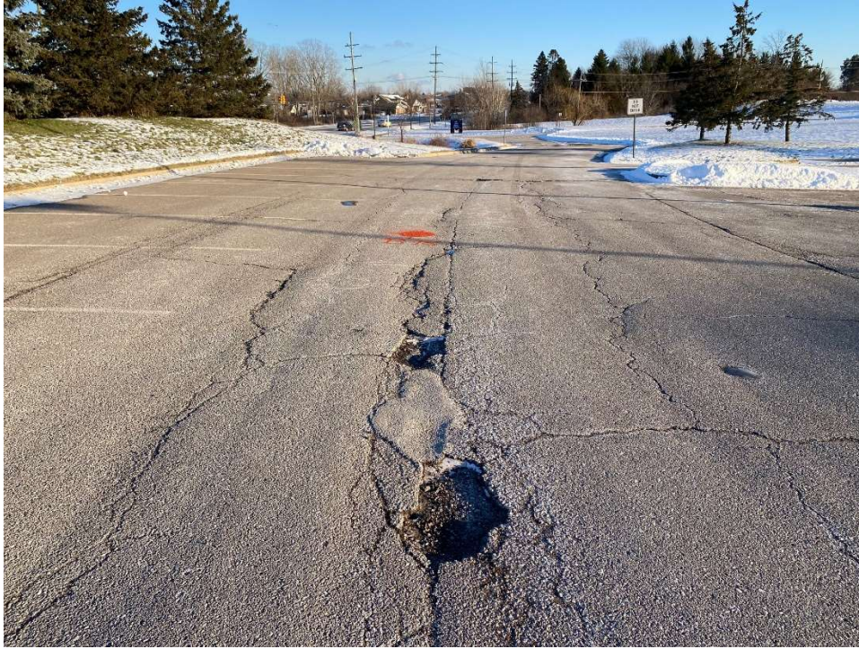
Photograph No. 15: Low to moderate severity transverse and longitudinal cracking with pot holes and cold patching at Mill Creek Middle School northeast parking lot near boring B-15. View to the east.
