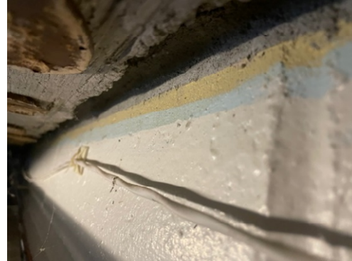
Figure 1 - Underside of Structural Slab
