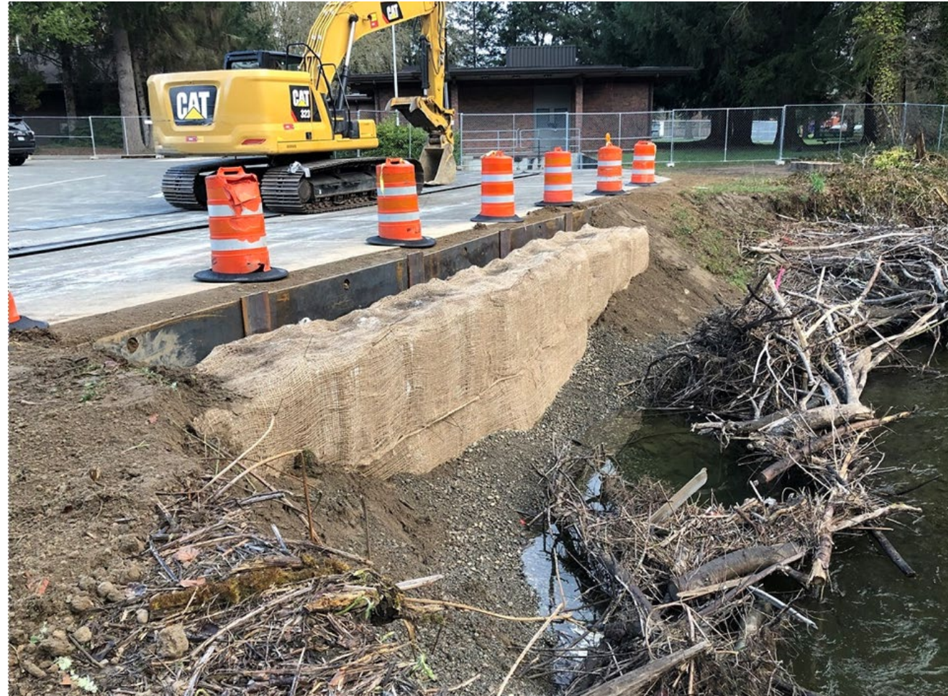
Temporary stream bank protection work completed
