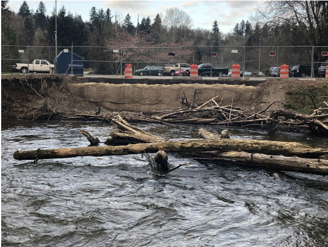
Temporary stream bank protection work completed
