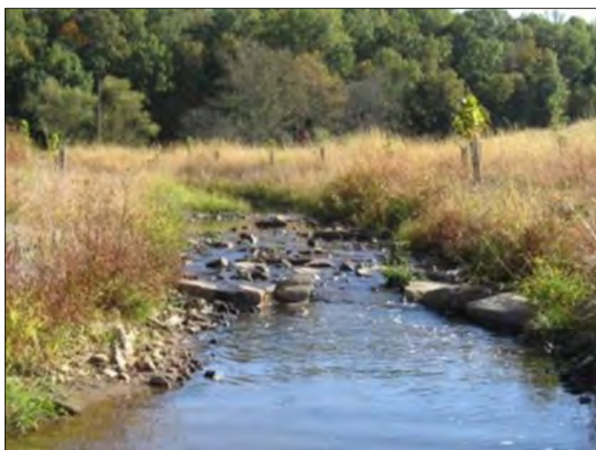
Figure 16: Constructed riffle
