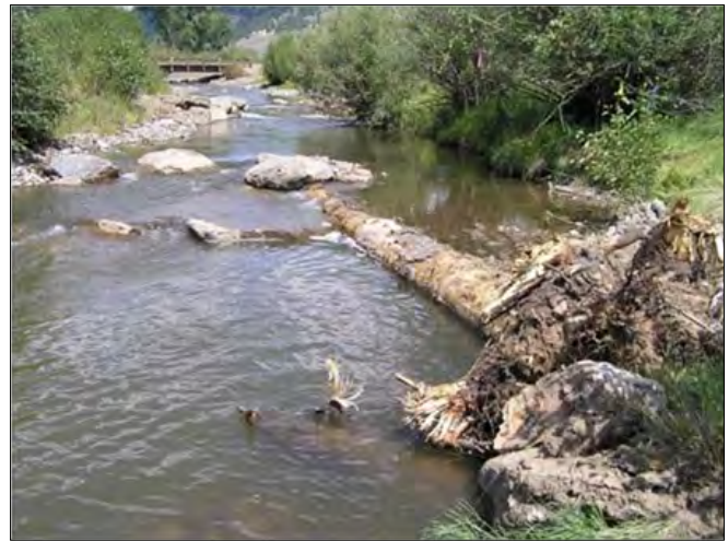
Figure 13: J-Hook log vane
