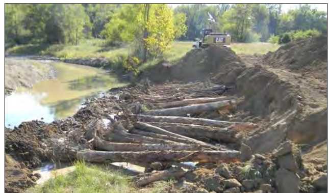
Figures 14 & 15: Wood toe structures
