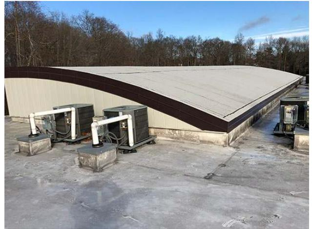
**Photo 18.** Media/computer wing with TPO membrane on low-slope roof and SBS roofing on barrel area
