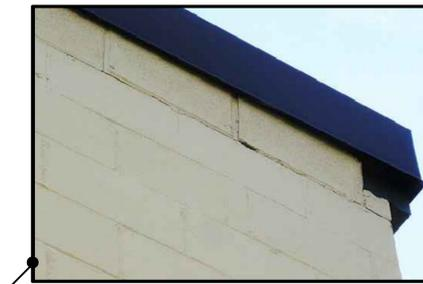
PHOTO 18: TYPICAL MASONRY DISPLACEMENT ALONG ROOF LINE.
