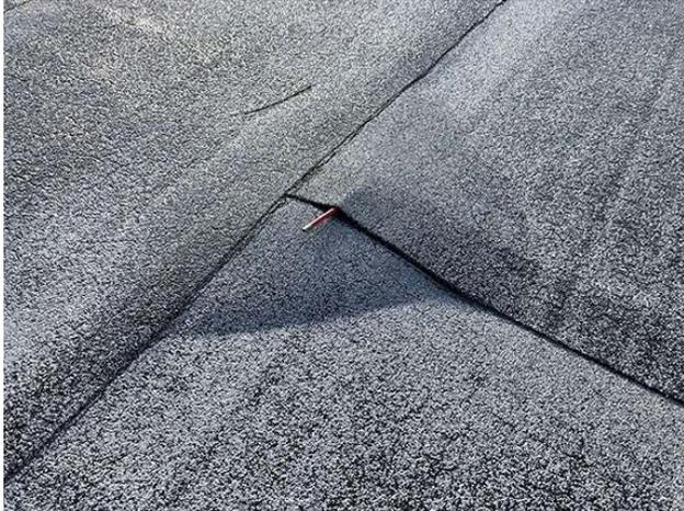
**Photo 19.** Typical blister in SBS roofing membrane
