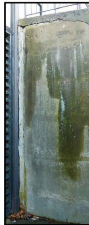
PHOTO 23: WIDENING OF CONTROL JOINT INDICATES MOVEMENT AND/OR SETTLING, TYPICAL ADJACENT TO BUILDING.
