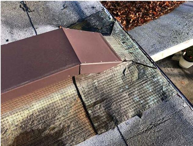
**Photo 7.** Expansion joint with aluminum cover - joint does not continue to roof edge
