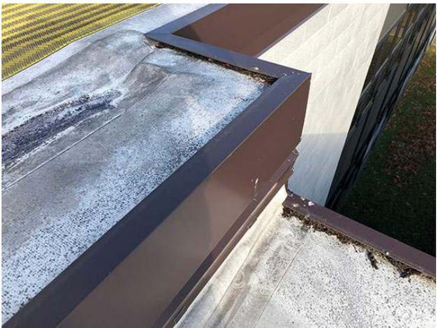
**Photo 17.** Aluminum fascia for single-ply membrane roofing
