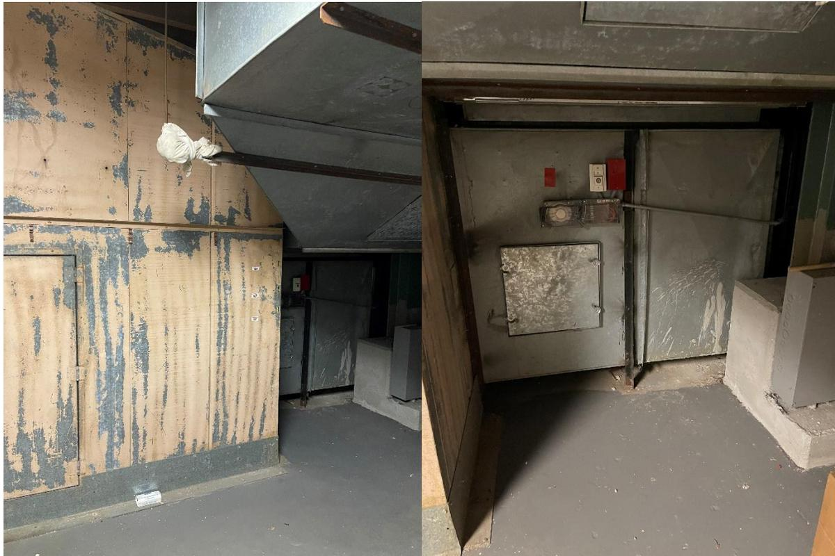
*Central Station Air Handler (S-1) and duct mounted smoke detector*
