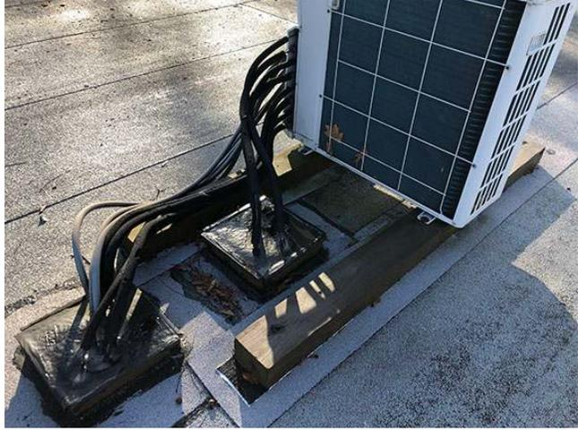
**Photo 10.** Typical pitch box and condensate unit
