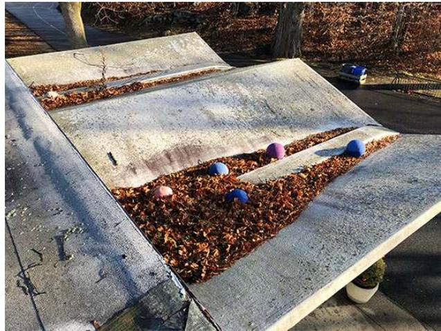
**Photo 8.** Sawtooth roof at entry with liquid roofing
