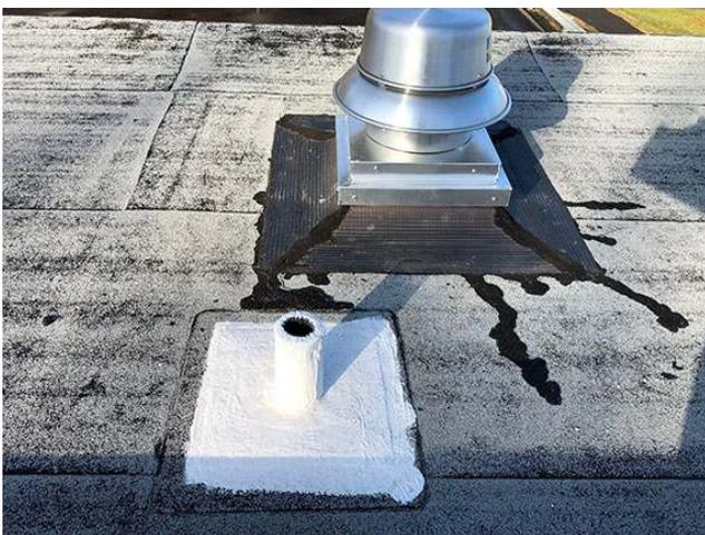
**Photo 11.** Typical rooftop fan unit and stack vent
