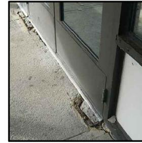
PHOTO 5: TYPICAL DETERIORATION AT DOOR THRESHOLDS.
