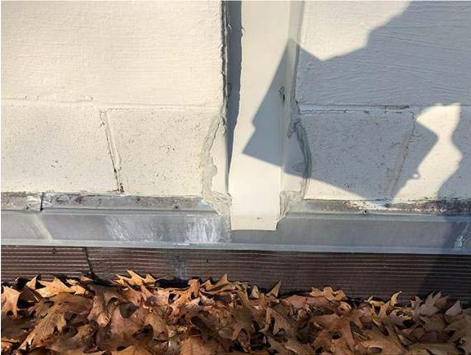
**Photo 25.** Base flashing detail along Auditorium wall with cover plate added to recess
