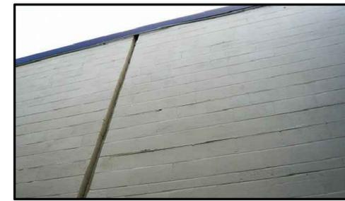
PHOTO 17: GROUT DISPLACEMENT OVER LARGE AREAS INDICATE MOVEMENT IN MASONRY.
