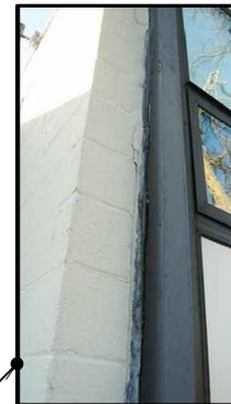
PHOTO 13: TYPICAL EXAMPLE OF JOINT SEALANT FAILURE BETWEEN STEEL STRUCTURE AND MASONRY. NOTE EVIDENCE OF SPALLING AND MASONRY DETERIORATION.
