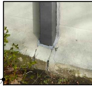
PHOTO 1: TYPICAL DETAIL AT BASE OF STEEL COLUMNS ALONG PERIMETER OF BUILDING. NOTE DETERIORATION OF CONCRETE AND REPAIRS USING SEALANT.
