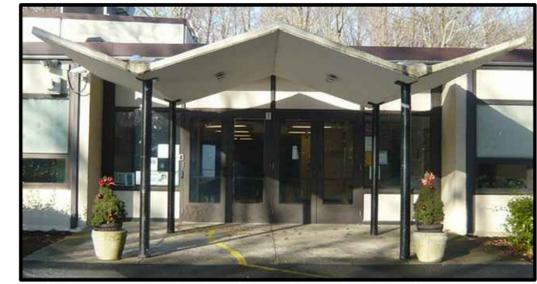
PHOTO 3: MAIN ENTRY CANOPY. NOTE LIQUID FLASHING MATERIAL APPLIED TO TOP SURFACE AND EVIDENCE OF WATER OVERFLOW AT EXPOSED EDGE OF CANOPY.
