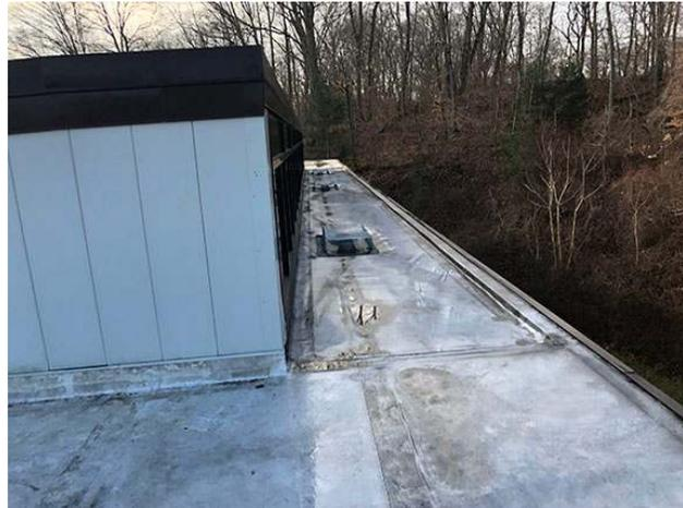
**Photo 20.** Metal siding on barrel roof and TPO single-ply membrane on low-slope roof
