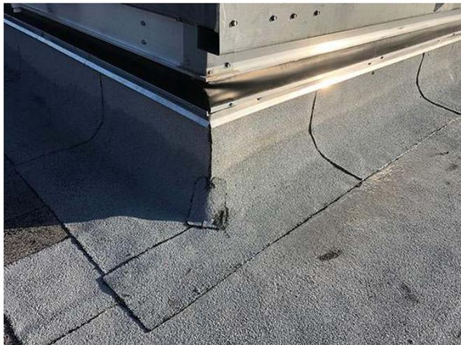
**Photo 3.** Roof Top Unit (RTU) base flashing using SBS membrane
