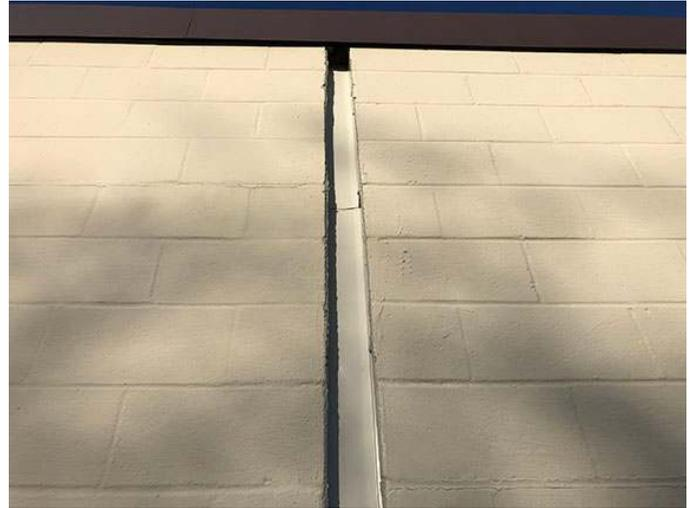
**Photo 26.** Roof line showing cover plate added to recess in Auditorium wall
