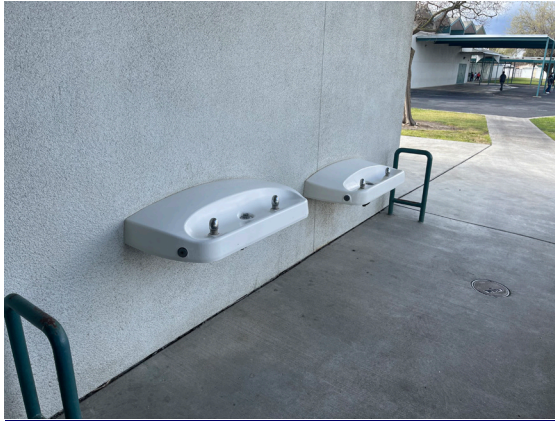
Replace drinking fountains with ADA compliant stations
