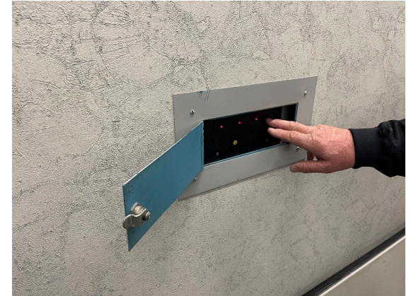
Remove lighting control relay switches, direct switch all new lights
