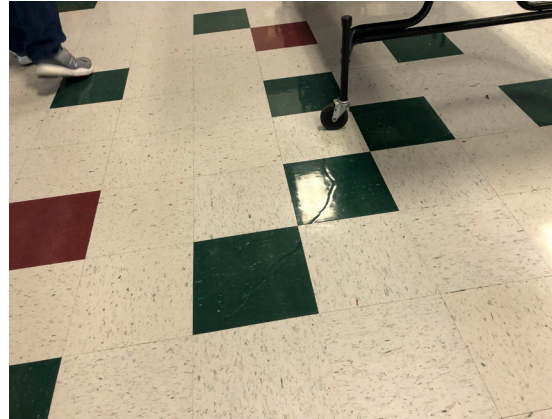
Replace multipurpose room VCT flooring
