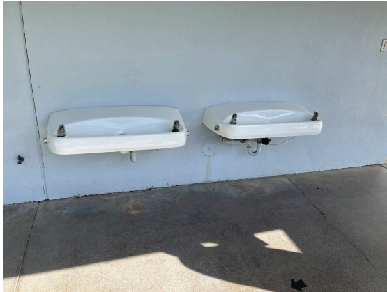
Replace drinking fountains with ADA compliant stations
