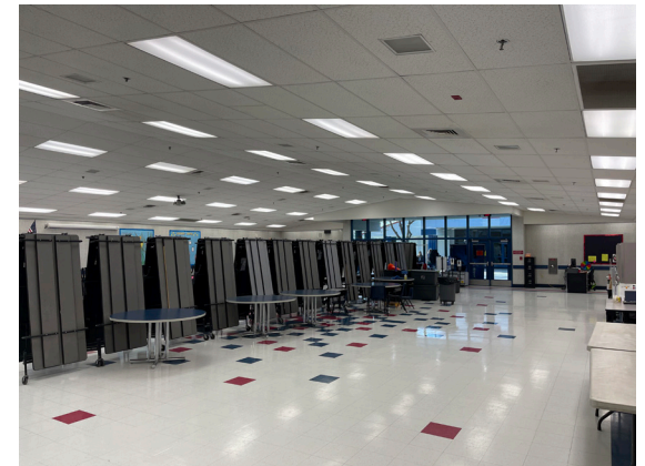
Replace multipurpose room VCT with LVT floor
