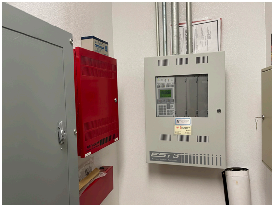
Replace fire panel and initiation devices
