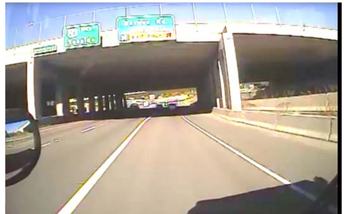
Off Ramp @ Barnes & HWY 217 North @ 15:09:21
