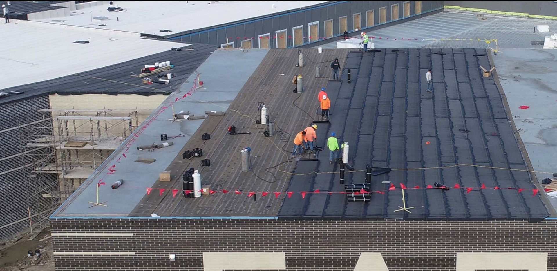
Intermediate School South: Modified Bitumen Roofing Layers Installation of the Base and Torch Sheets
