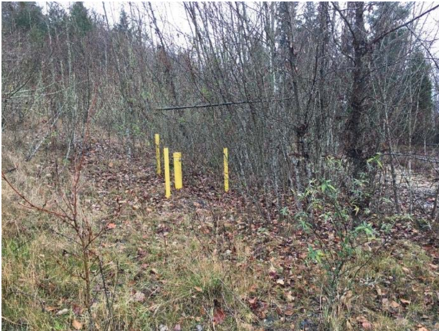
6. LOOKING NORTH ON THE NORTHERN PORTION OF THE SUBJECT PROPERTY AT ONE OF THE MONITORING WELLS OBSERVED ON THE SUBJECT PROPERTY. LIGHT VEGETATION AND IMMATURE TREES WERE OBSERVED HERE.
