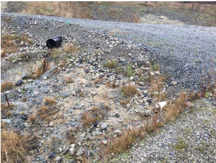
4. LOOKING NORTHWEST NEAR THE NORTH ENTRANCE OF THE SUBJECT PROPERTY AT 12-INCH STORMWATER OUTFALL PIPES.
