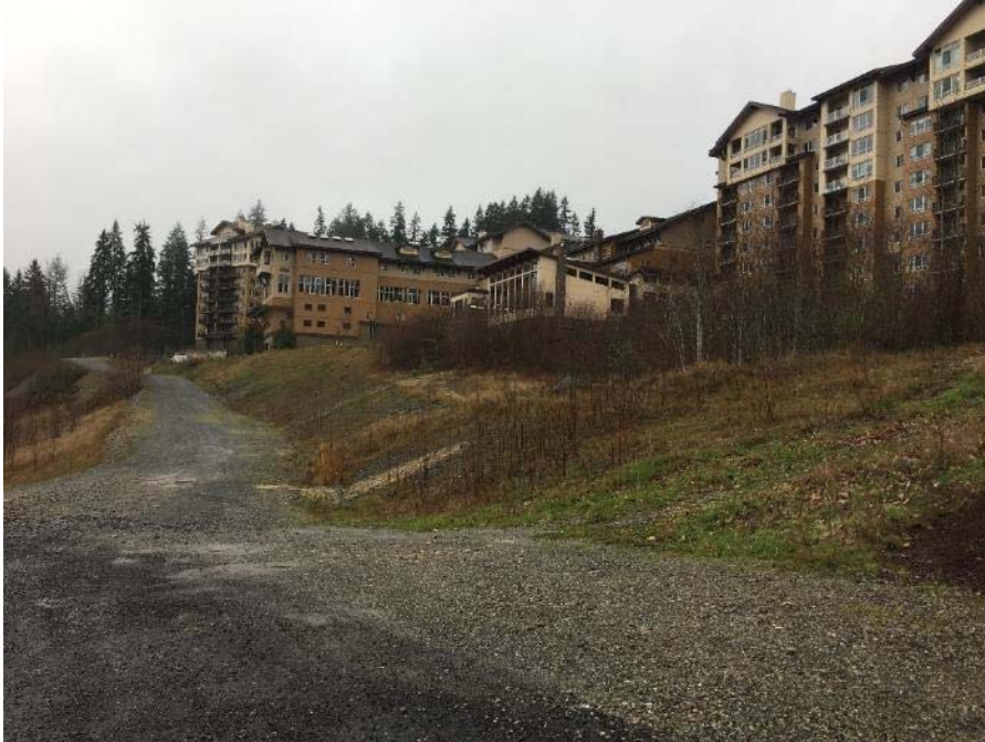
5. LOOKING SOUTH-SOUTHWEST FROM NORTH ENTRANCE OF SUBJECT PROPERTY AT ACCESS ROAD ON THE WESTERN PORTION OF THE SUBJECT PROPERTY AND THE WEST-ADJACENT SENIOR LIVING FACILITY.
