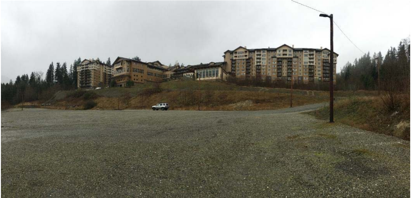
9. LOOKING WEST-SOUTHWEST FROM THE NORTHEAST END OF GRAVEL PAD AREA WITH A PANORAMIC VIEW OF THE WEST HALF OF THE SUBJECT PROPERTY AND THE WEST-ADJOINING PROPERTY.
