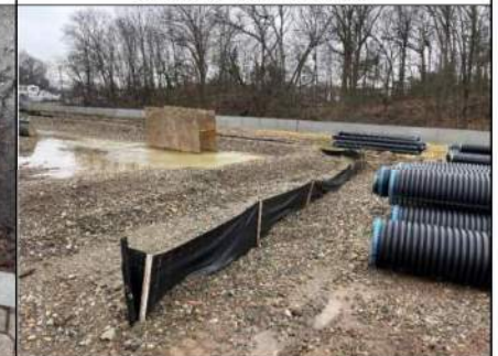
Condition of temporary sediment trap in south of site
