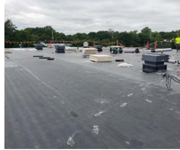
Freshman Center Roof
