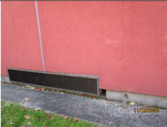
Unit ventilator in place at ground level. Cold air and surface water have an open pathway into the building.
