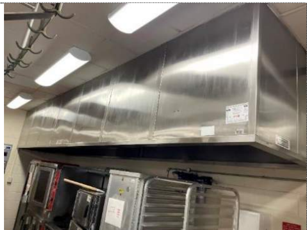
Figure 11: Kitchen exhaust hood.
