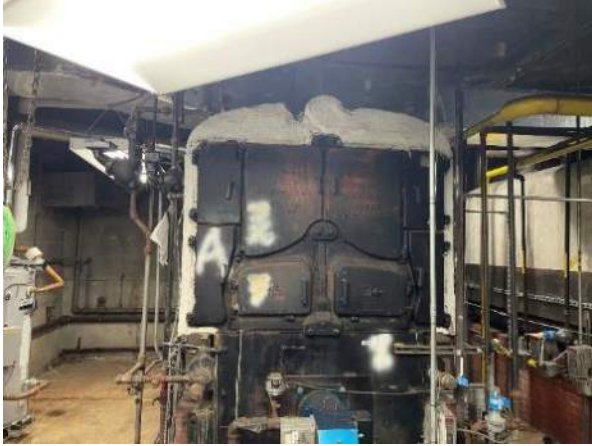
Figure 3: Steam boilers original to the building (cr 1953).
