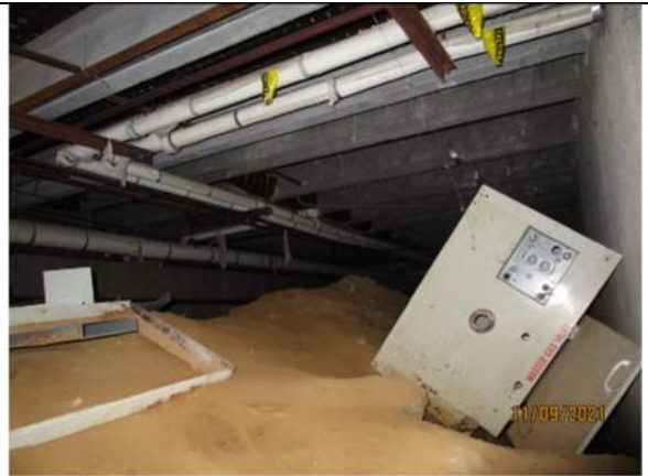
Soils with no vapor barrier allow moisture vapor from the ground into the building.
