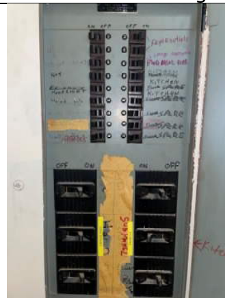
Figure 18: Old FPE panel outside the boiler room
