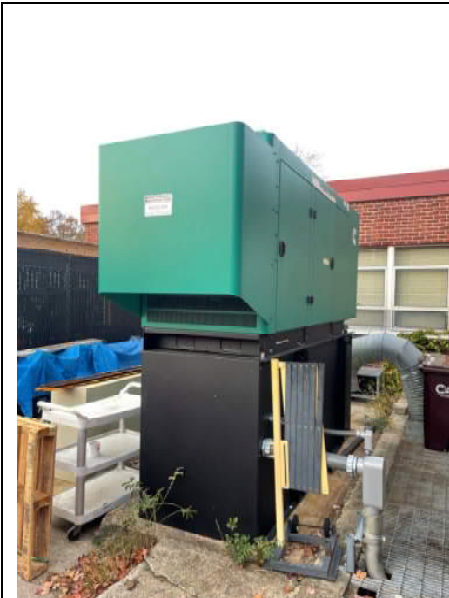
Figure 21: New 125kW Cummins emergency generator
