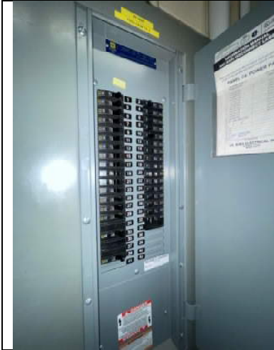
Figure 13: Newer Square D panel serving the 200 wing
