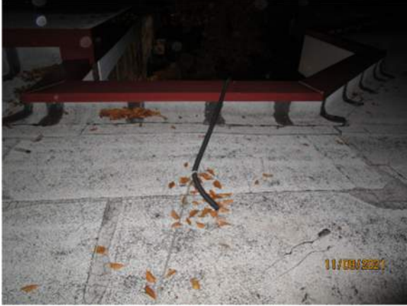
The sump pump discharges onto the roof as there is no drain in the courtyard.
