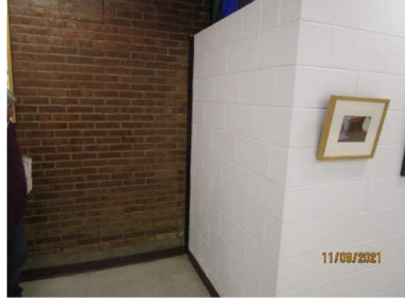
This corner near the ramp is where the water was actively observed entering the building.
