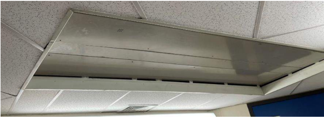
Figure 9: Four-Pipe Fan Coil Unit.
