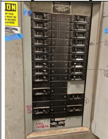
Figure 15: Old FPE panel serving the kitchen area
