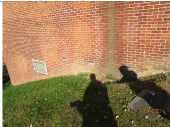
The masonry wall extends below grade with no apparent foundation or waterproofing membrane.
