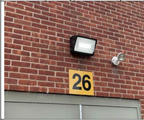
Figure 25: Exterior LED WallPak fixture
