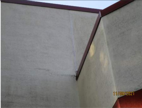
Cracks in the finish system have been sealed to try to prevent water infiltration.
