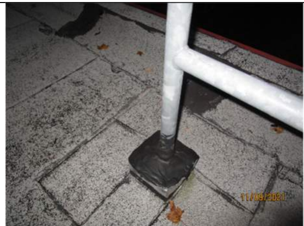
Pitch box at the guardrail has been refreshed.
