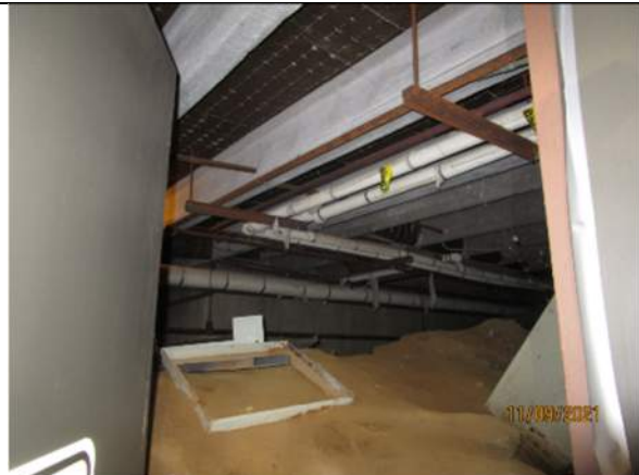
Soils with no vapor barrier allow moisture vapor from the ground into the building.
