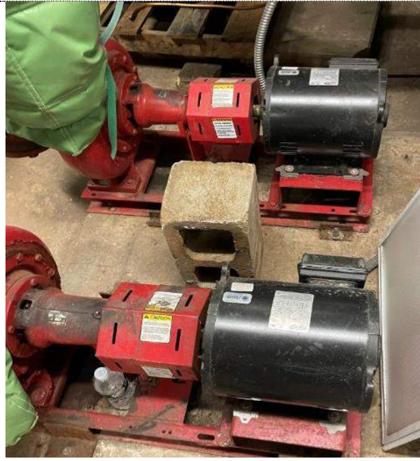
Figure 6: Heating HW pumps in boiler room
