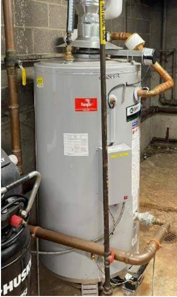
Figure 12: AO Smith 120MBH domestic hot water heater.
