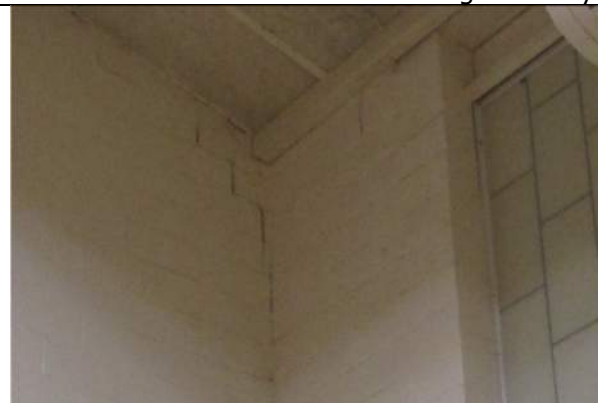
Cracks in the gym wall up to the roof level. Cracking in the masonry wall in the gym at the roof line.
