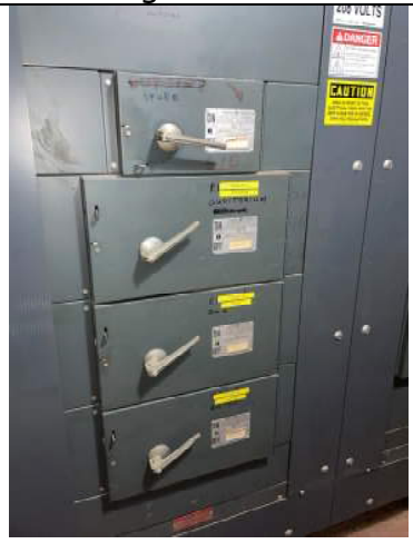
Figure 16: Older General Electric switchboard serving 100 wing
