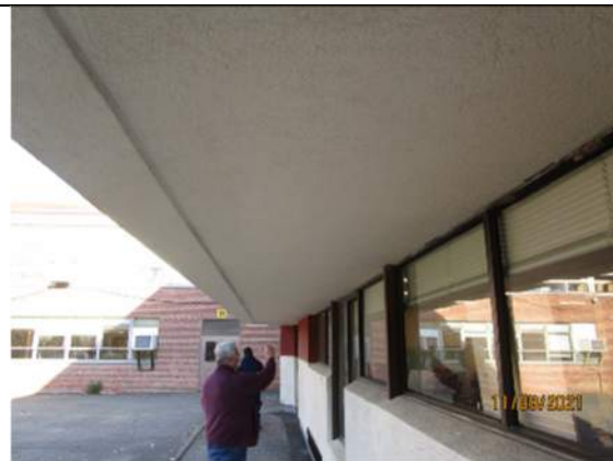
Little to no ventilation in the soffits.
