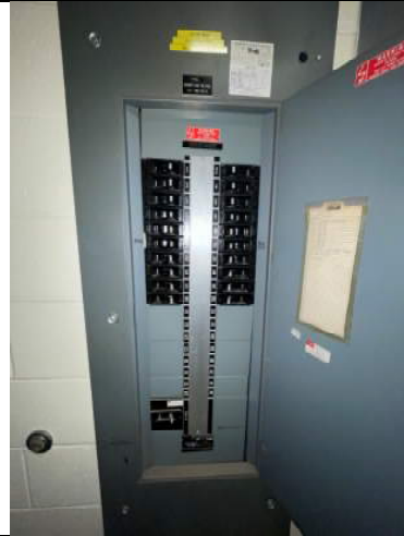
Figure 14: Old FPE panel serving the 200 wing
