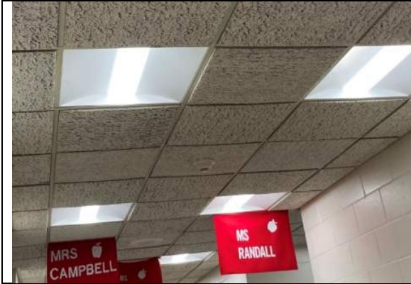
Figure 23: Recessed LED fixtures in classrooms, library, and office spaces
