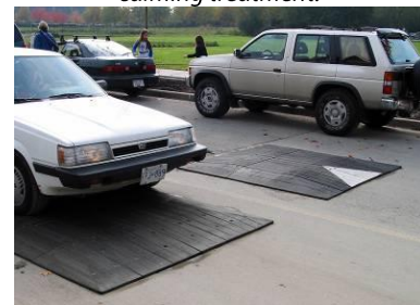
Speed lumps or cushions are divided to allow emergency vehicles to pass unaffected.
