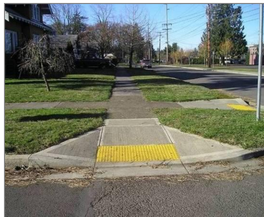
Example of an ADA-compliant perpendicular curb ramp.
