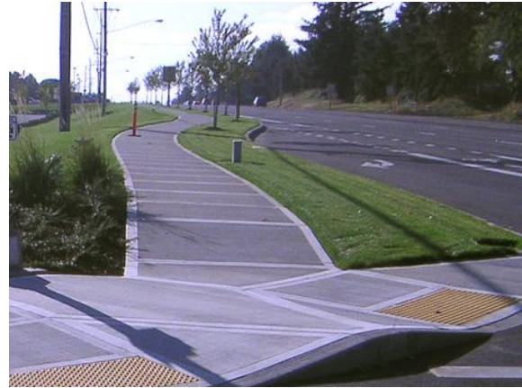
The ideal condition along most sections of US Route 1 would be a 6' sidewalk with a grassy strip separating pedestrians from traffic.
