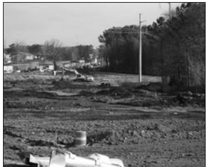
Figure 2. Construction of new buildings and roads disturbs the native soil.
