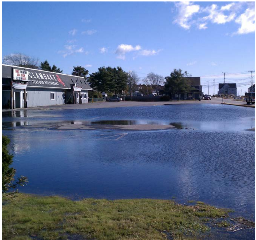
Flooding in Scarborough during king tide
