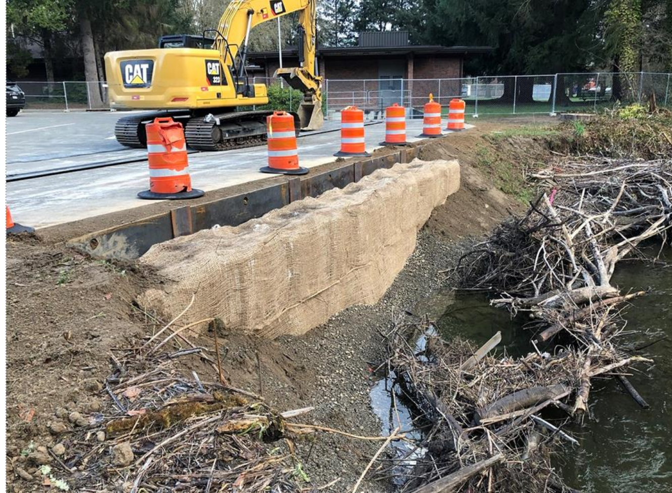
Temporary stream bank protection work completed
