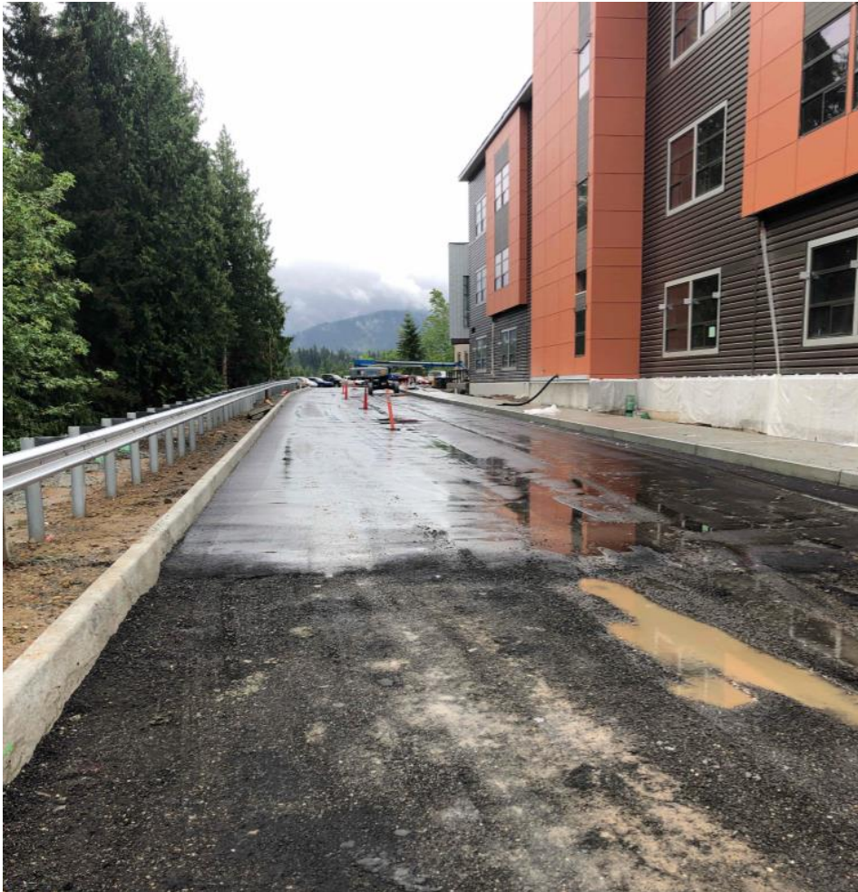
Main drive along north side of the building paved with first layer of ATB
