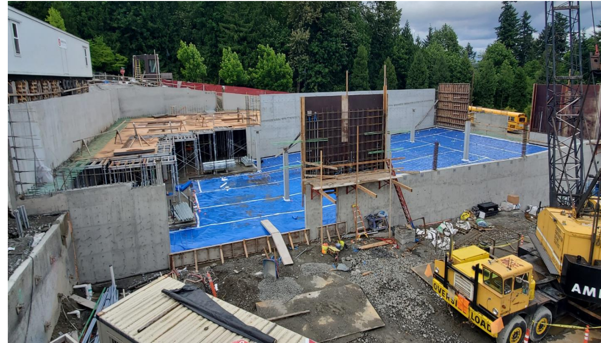
Foundation walls for the parking garage in place and forming for the 2 nd level deck being placed
