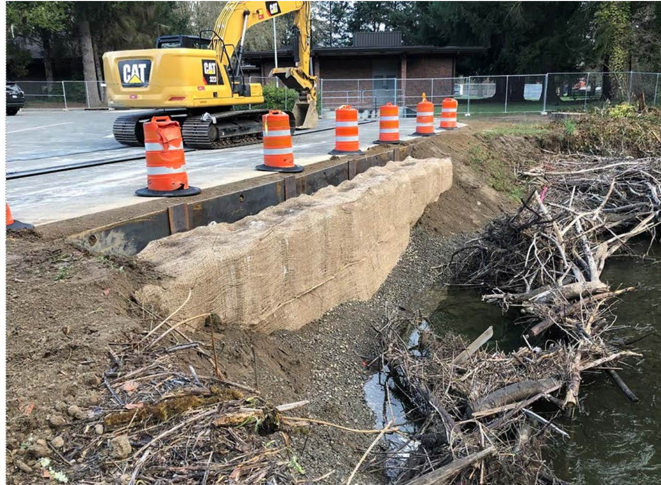
Temporary stream bank protection work completed
