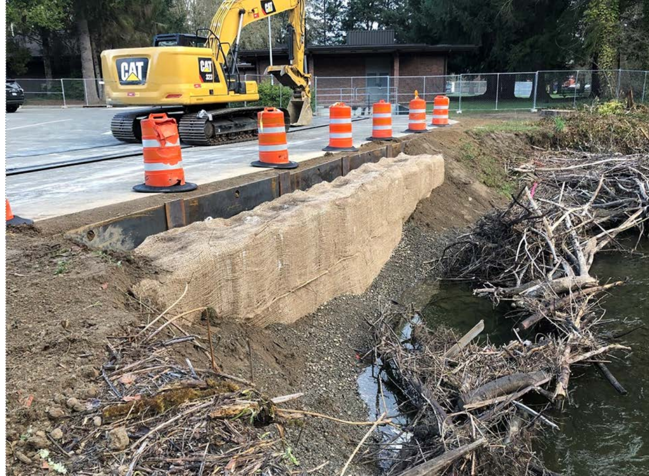
Temporary stream bank protection work completed
