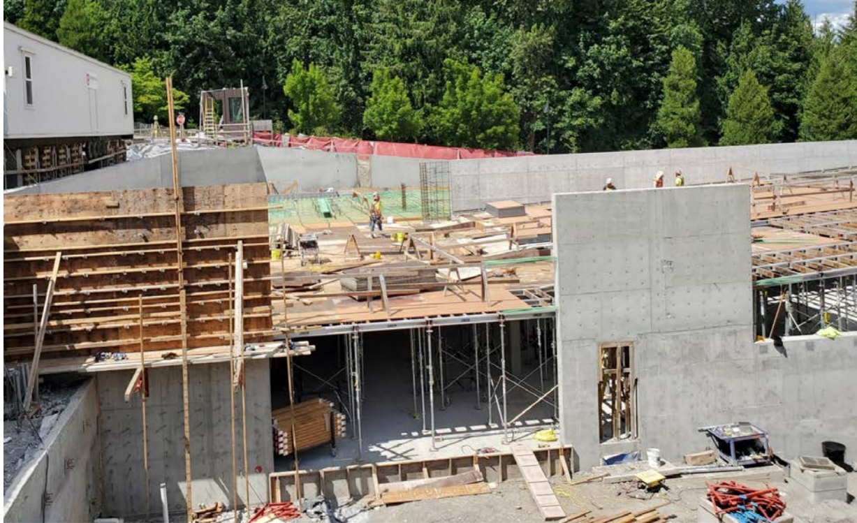
Top level of the parking garage be prepped & formed for concrete pour
