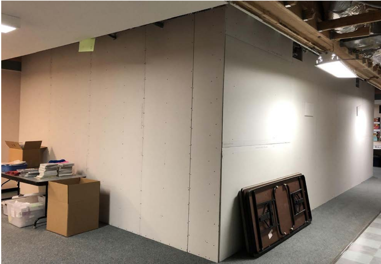
Framing and sheetrock for new offices in pod area underway
