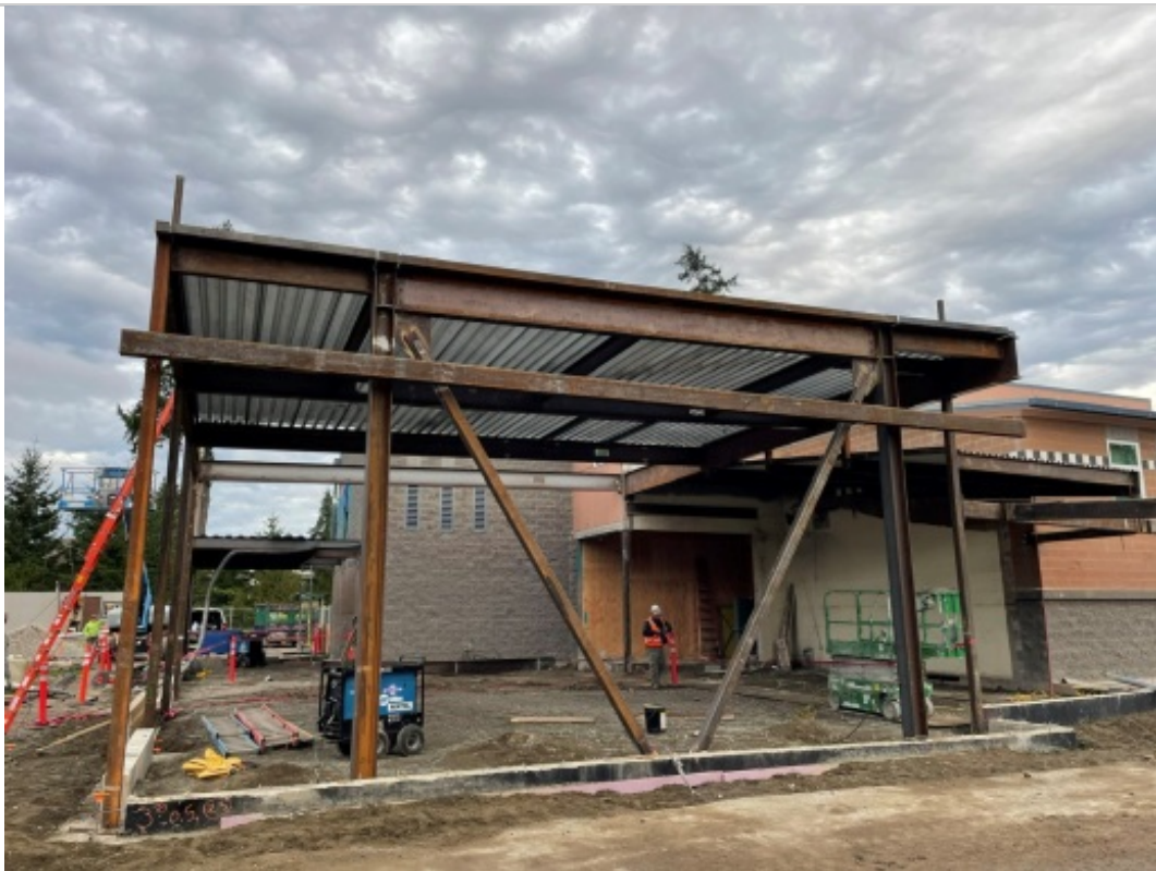
Steel structure complete and roof decking installed for expanded commons area:
