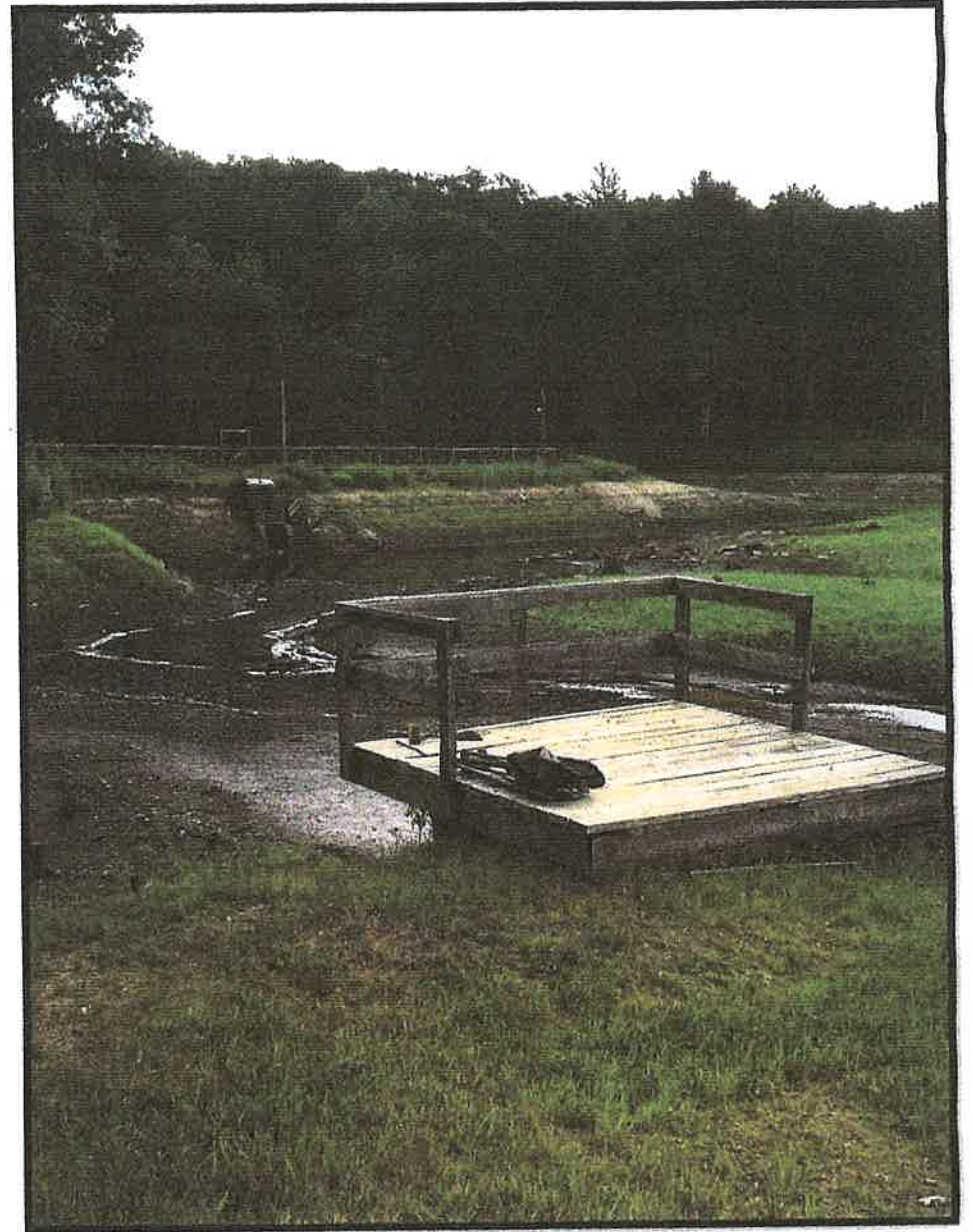
Summer 2020 The earthen dam looks solid from the water side and on the top surface. The outer bank is where shallow sink holes have appeared indicating the internal erosion. A video camera inserted through the valve pipe and sample core borings from the top down have disclosed the sand and gravel content of the interior structure is not the correct material, it does not contain the necessary amount of clay for sustainability.
