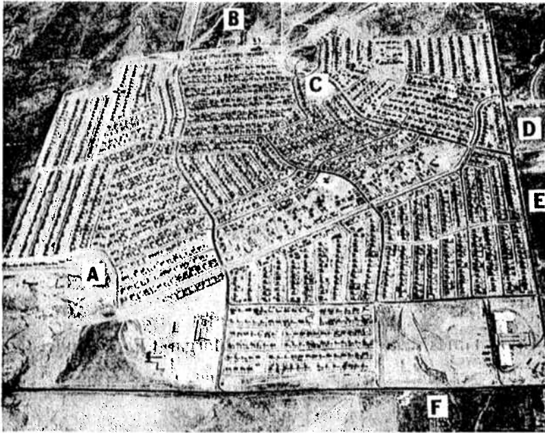
On October 16, 1956, the Thornton Tribune featured this photograph, documenting the continuing growth of Thornton. A The new city hall. B New residential section of the city. C Bertha Heid Elementary School. D Dream House Acres. E City View Heights. F New shopping centers on North Washington.
