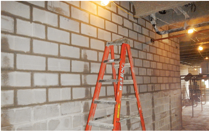
Interior CMU walls being constructed at the High School Team Room Addition.
