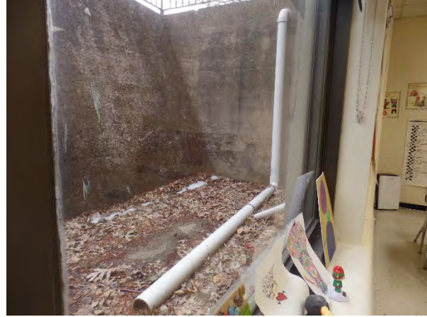
Exterior drainage slopes to building at below grade rooms Areaways fill with debris causing flooding
