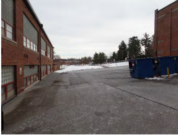
Exterior drainage slopes to building at below grade rooms Areaways fill with debris causing flooding
