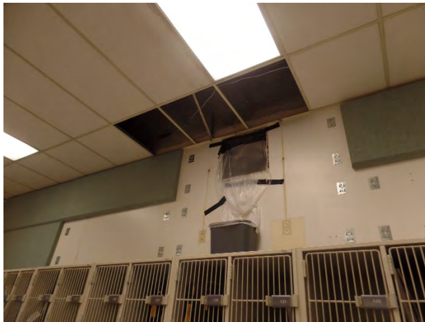
Active Roof Leak
