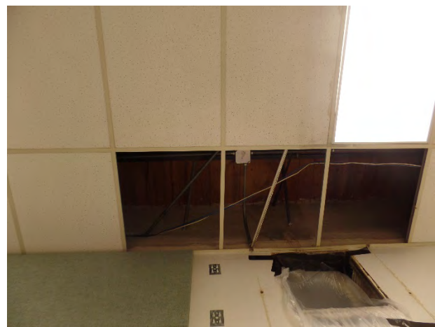
Active Roof Leak
